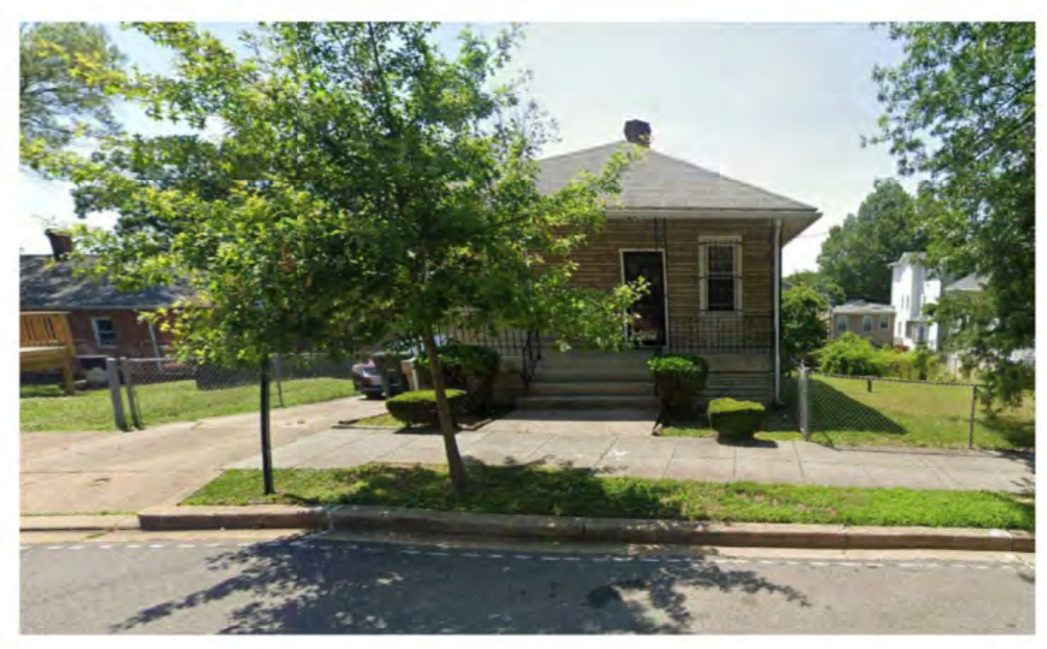
VIEW FROM 57TH STREET
