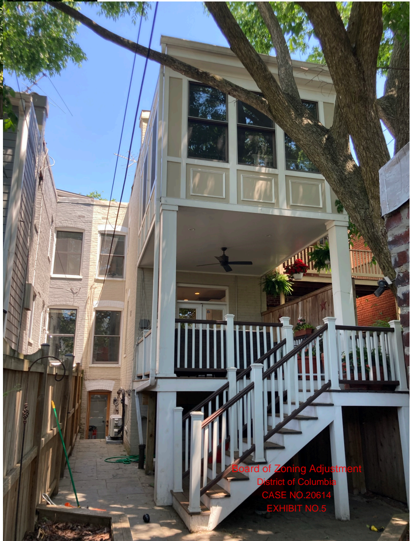
EXISTING REAR FACADE
