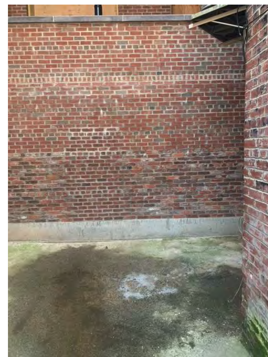
SOUTH PROPERTY LINE AT NEW DEVELOPMENT WALL
