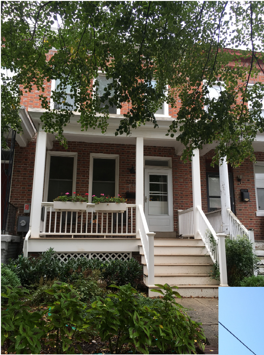
FRONT FAÇADE, 1322 D STREET SE
