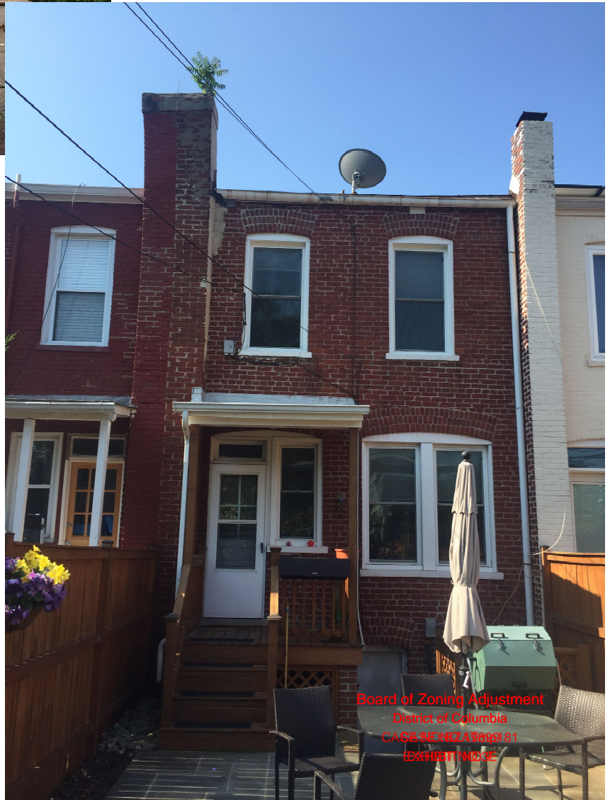
EXISTING REAR FACADE
