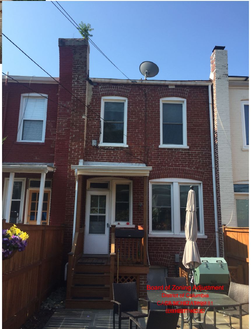
EXISTING REAR FACADE
