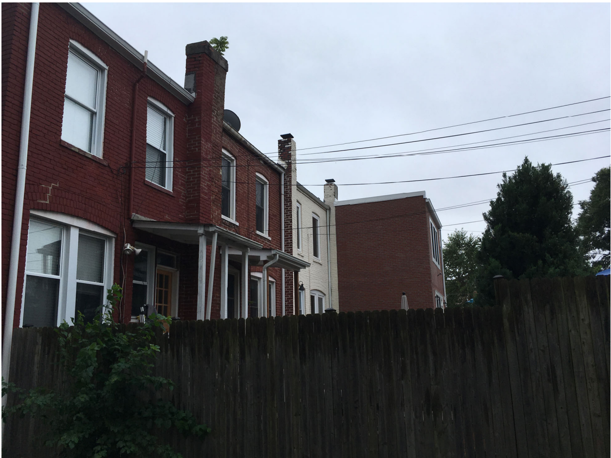
REAR VIEW FROM SIDE ALLEY (LOOKING EAST)
