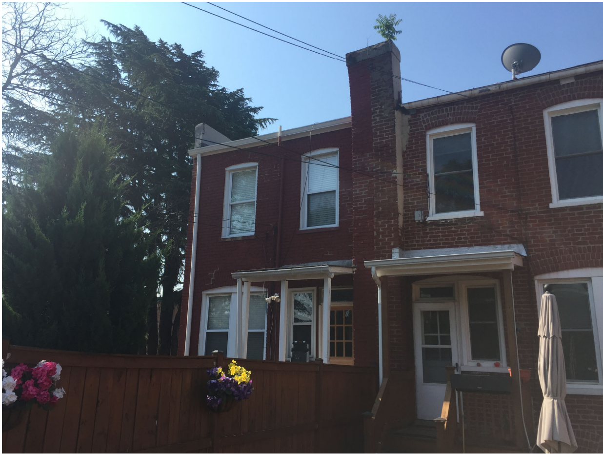
REAR VIEW LOOKING WEST
