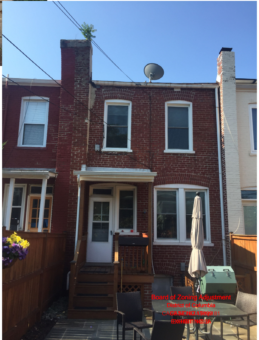
EXISTING REAR FACADE
