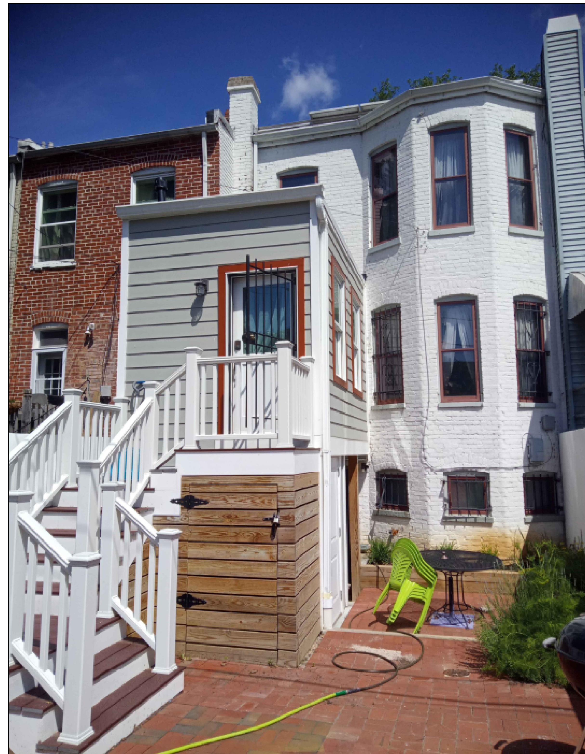
3 EXISTING REAR YARD PHOTOGRAPH A001
