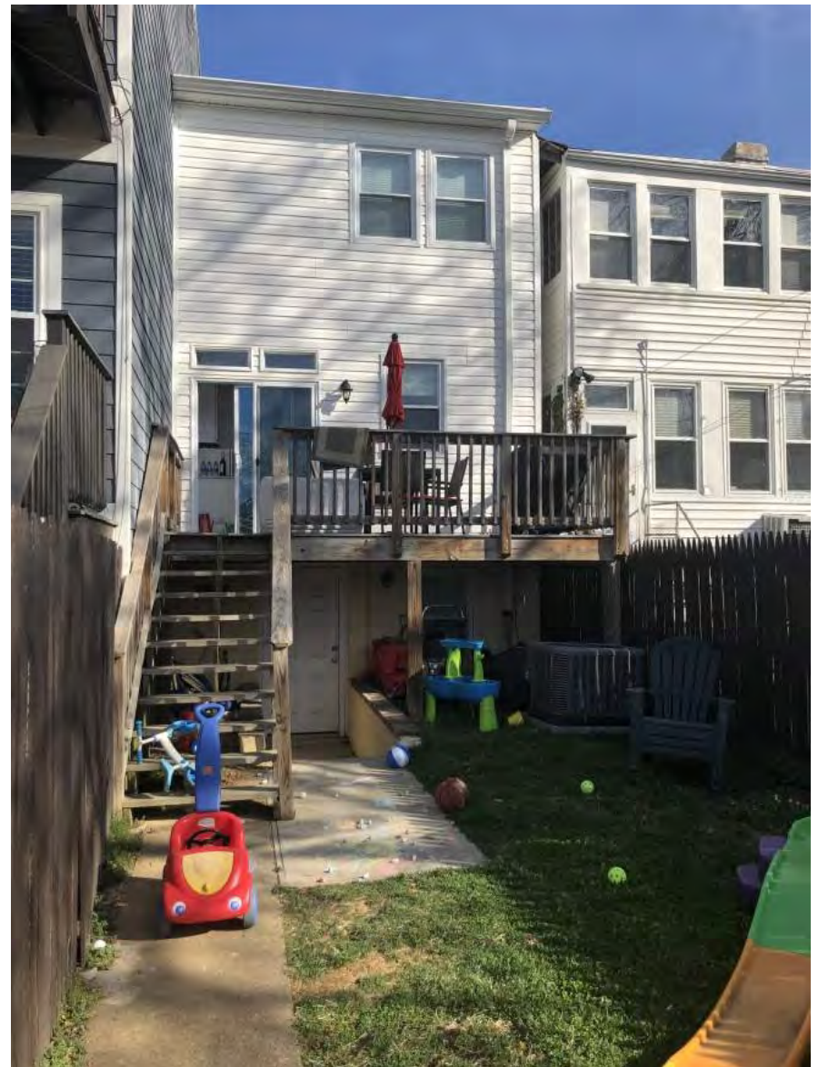
Rear Yard of Subj. Property Looking from the Alley
