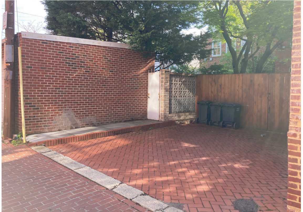
View of Property from the southwest
