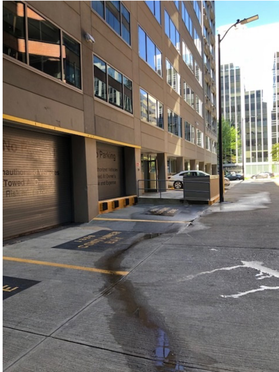
EXISTING BUILDING ALLEY AND NORTH ELEVATION LOOKING WEST TOWARD 19TH STREET
