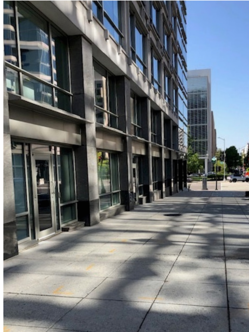
EXISTING BUILDING 19TH STREET NW LOOKING SOUTH
