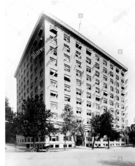
Commerce Building, 1831 H Street NW ~1920s
