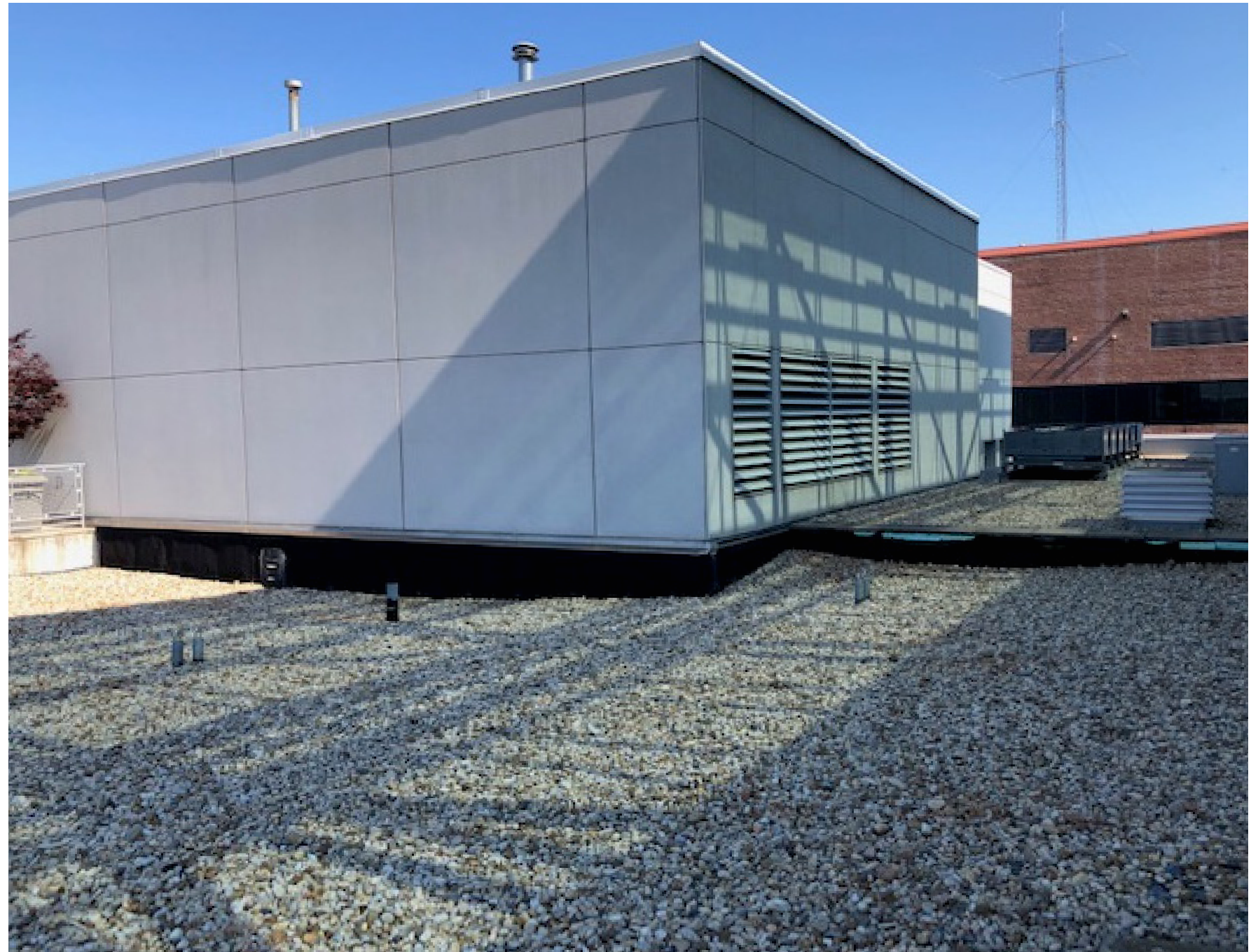
EXISTING PENTHOUSE SOUTHEAST CORNER LOOKING NORTHWEST
