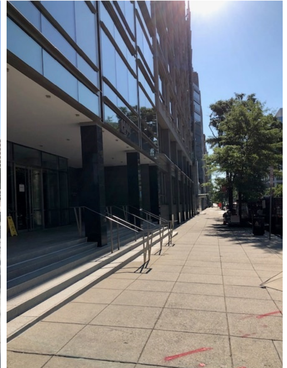
EXISTING BUILDING PENNSYLVANIA AVENUE / H STREET NW LOOKING EAST
