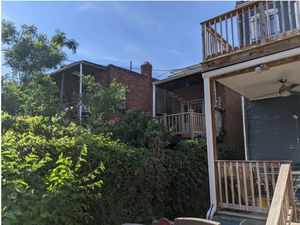
FROM REAR YARD LOOKING NW
