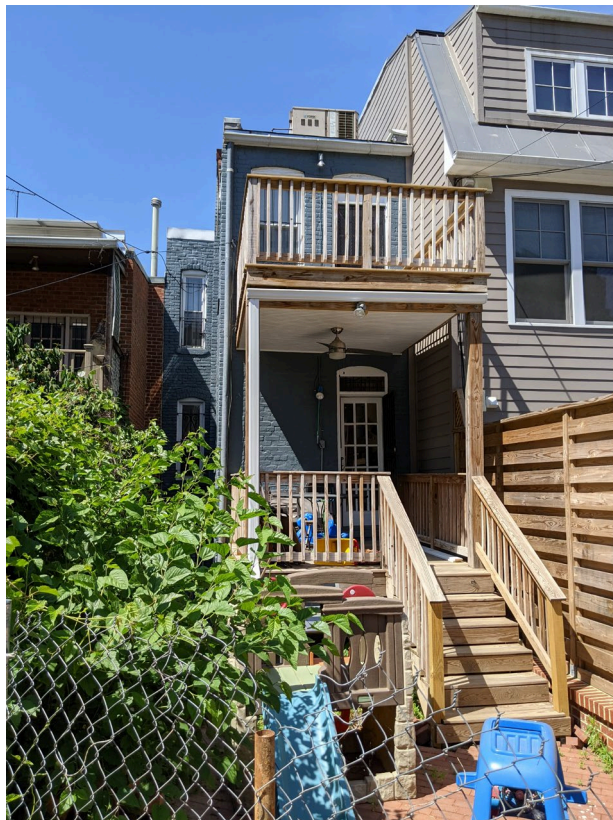
EXISTING REAR FACADE
