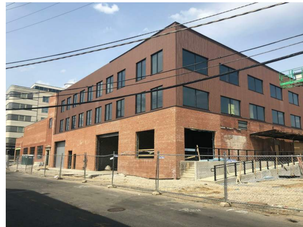
SIDE VIEW LOOKING NORTHEAST ALONG FENWICK STREET NE
