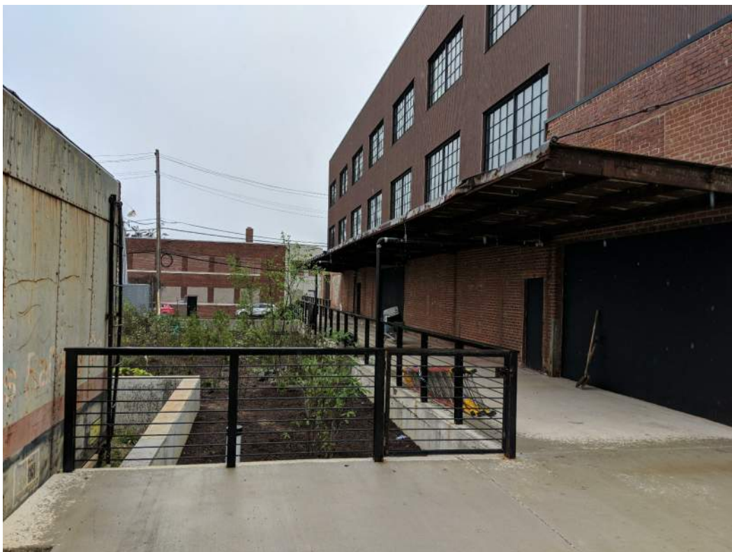
VIEW OF WEST BUILDING FROM TRAINCAR & PLAZA
