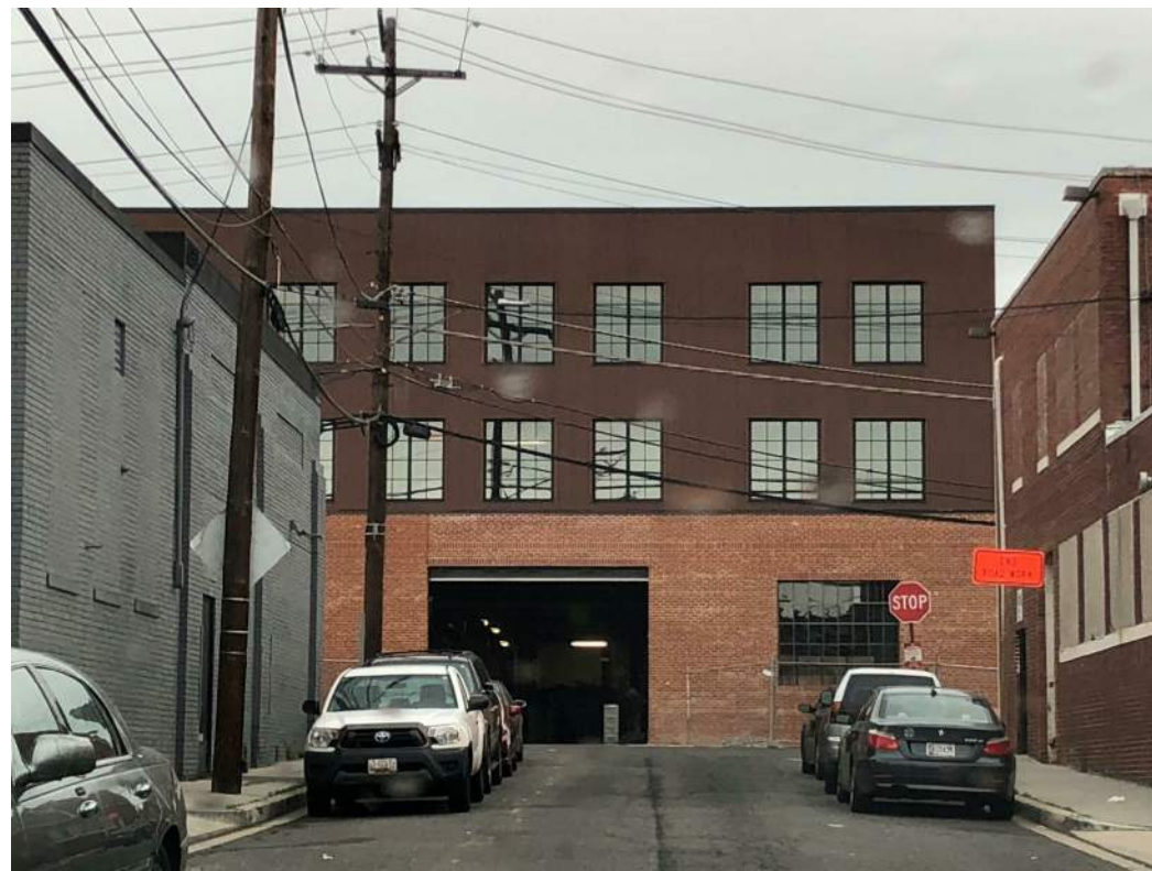
SIDE VIEW LOOKING EAST FROM GALLAUDET STREET NE
