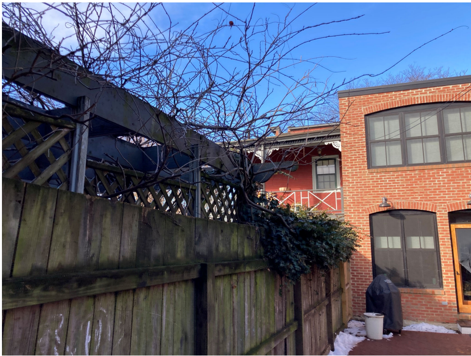
REAR FAÇADE, VIEW TO SOUTH
