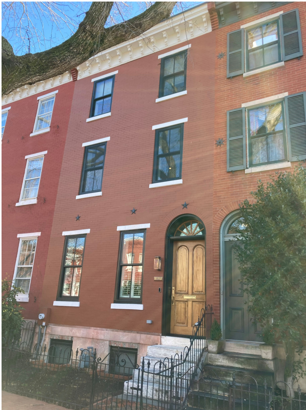
EXISTING FRONT FACADE
