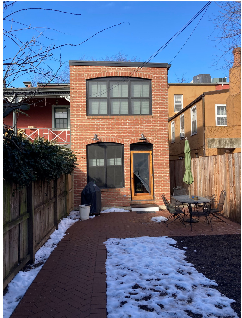
EXISTING REAR FACADE
