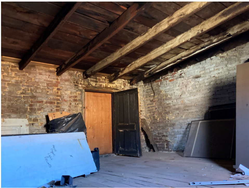
EXISTING GARAGE ATTIC
