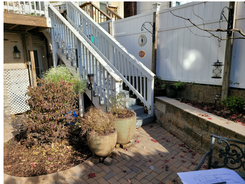
Image E: Existing stair landing
