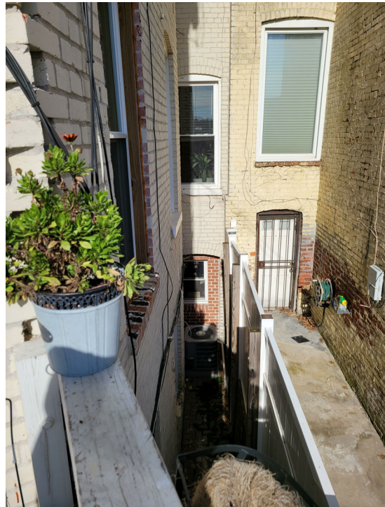
Image J: View of property line between subject property and adjacent property (14 Quincy PI NW)
