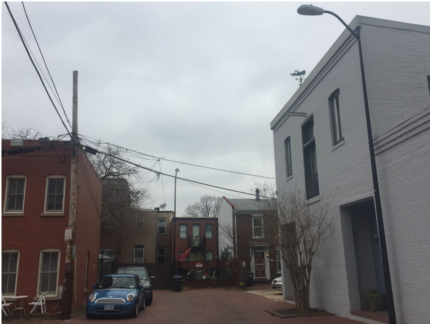
VIEW FROM ALLEY, FACING NORTH
