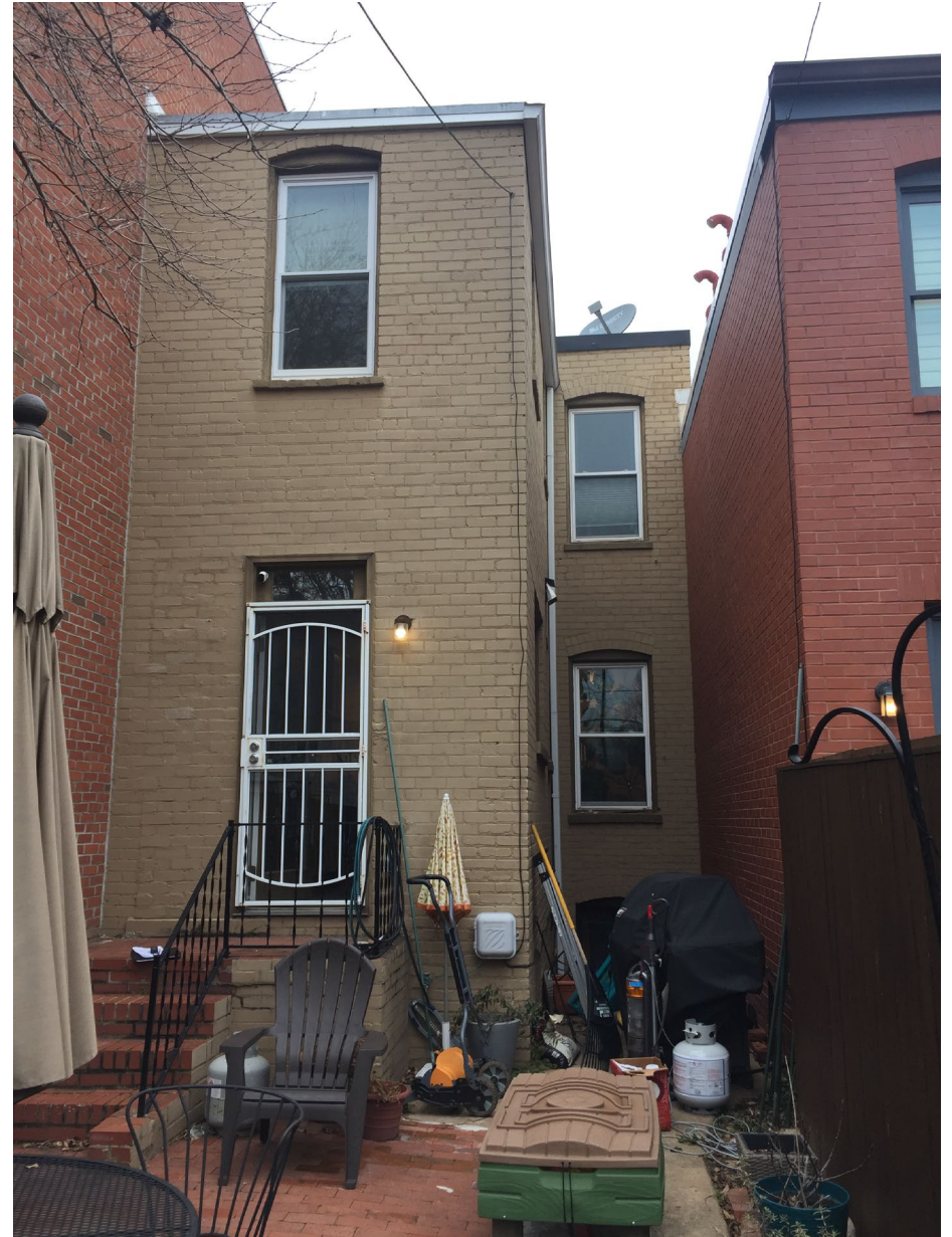
EXISTING REAR FACADE
