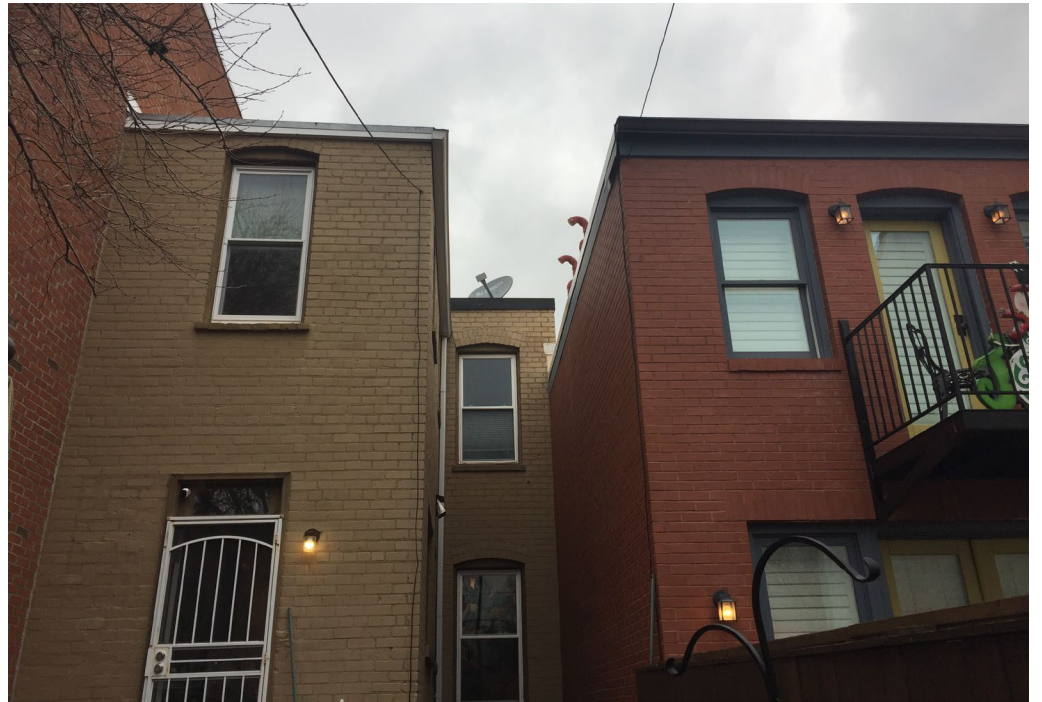
REAR FAÇADE, LOOKING EAST
