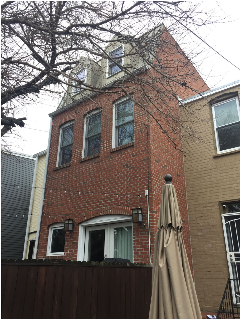
REAR FAÇADE, LOOKING WEST
