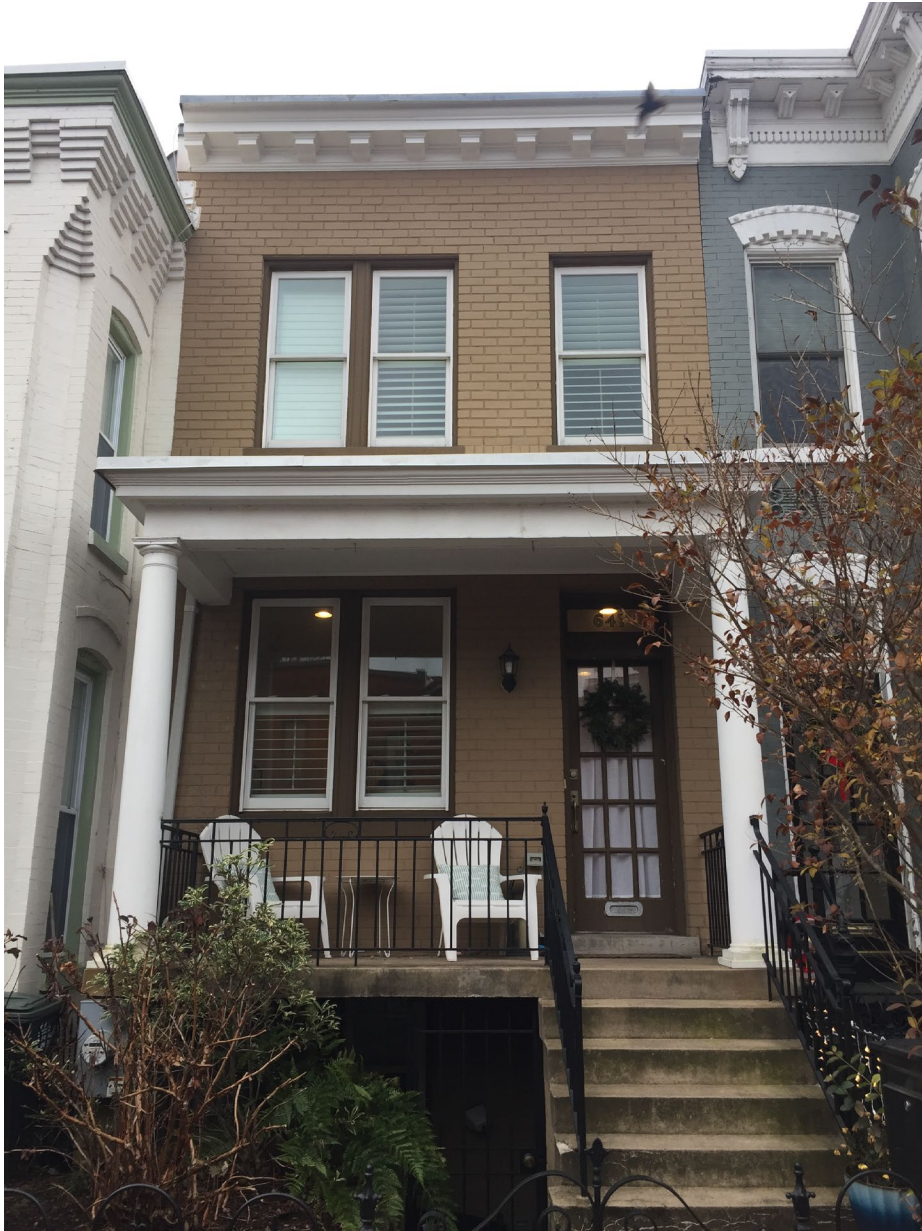
EXISTING FRONT FACADE
