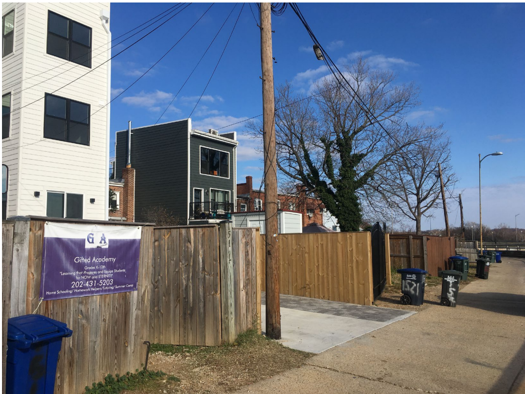
VIEW FROM ALLEY LOOKING NORTH-EAST
