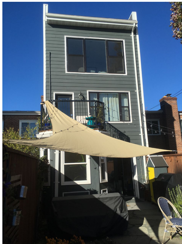
EXISTING REAR FACADE
