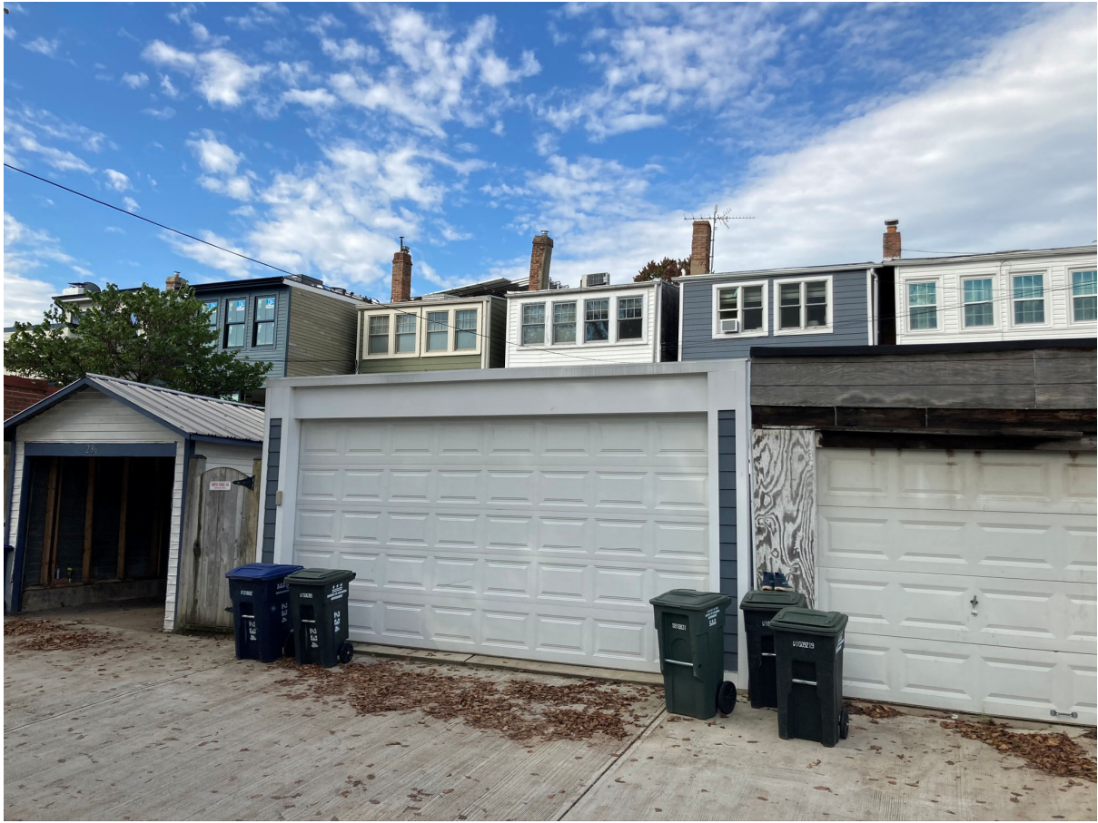
ALLEY NORTH VIEW
