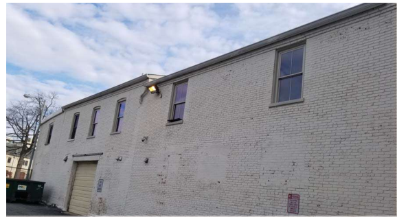
EXISTING SITE STRUCTURE
