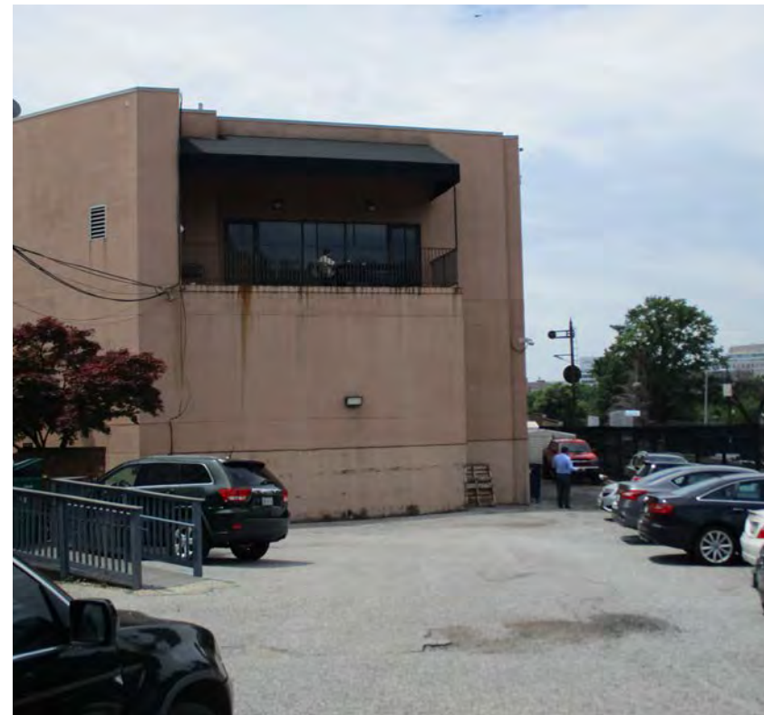
structure in alley to southwest
