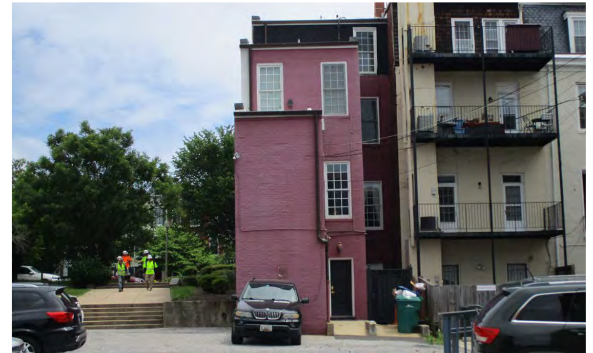
existing condition - alley view
