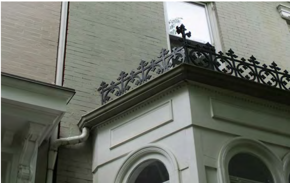
bay window detail
