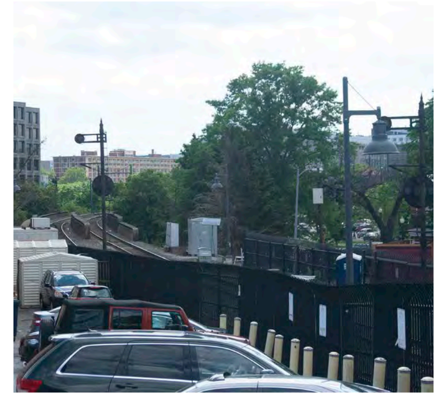
view southwest along railroad tracks
