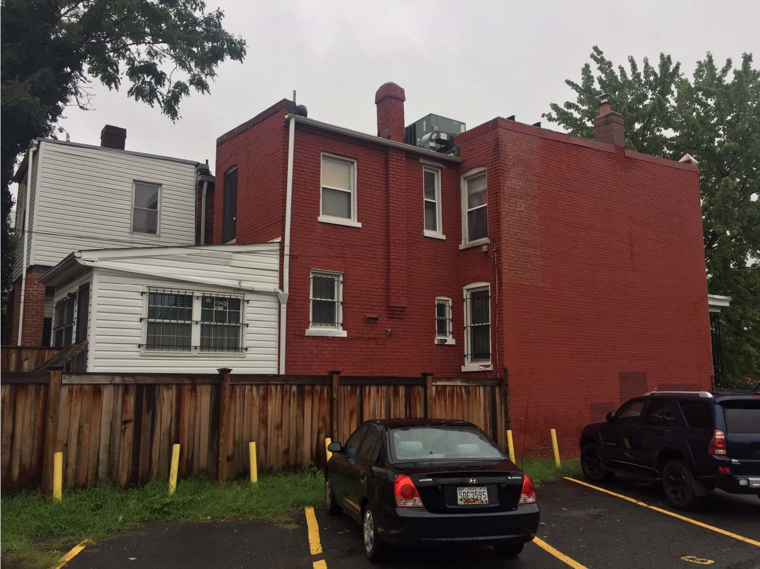
Side View from Adjacent Parking Lo
