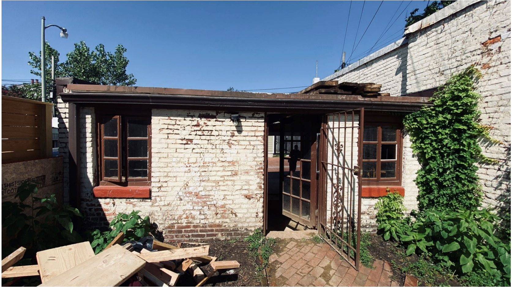
Garage façade / Yard view
