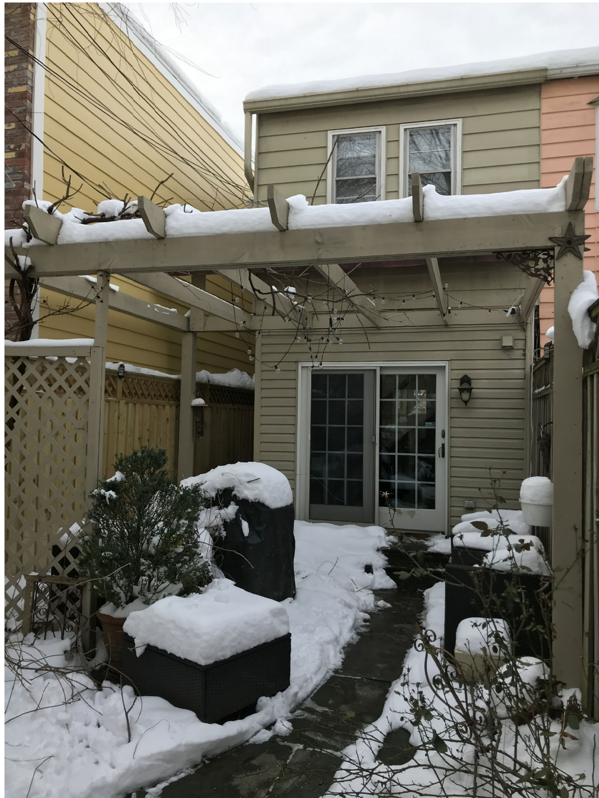
REAR VIEW, EXISTING ADDITION
