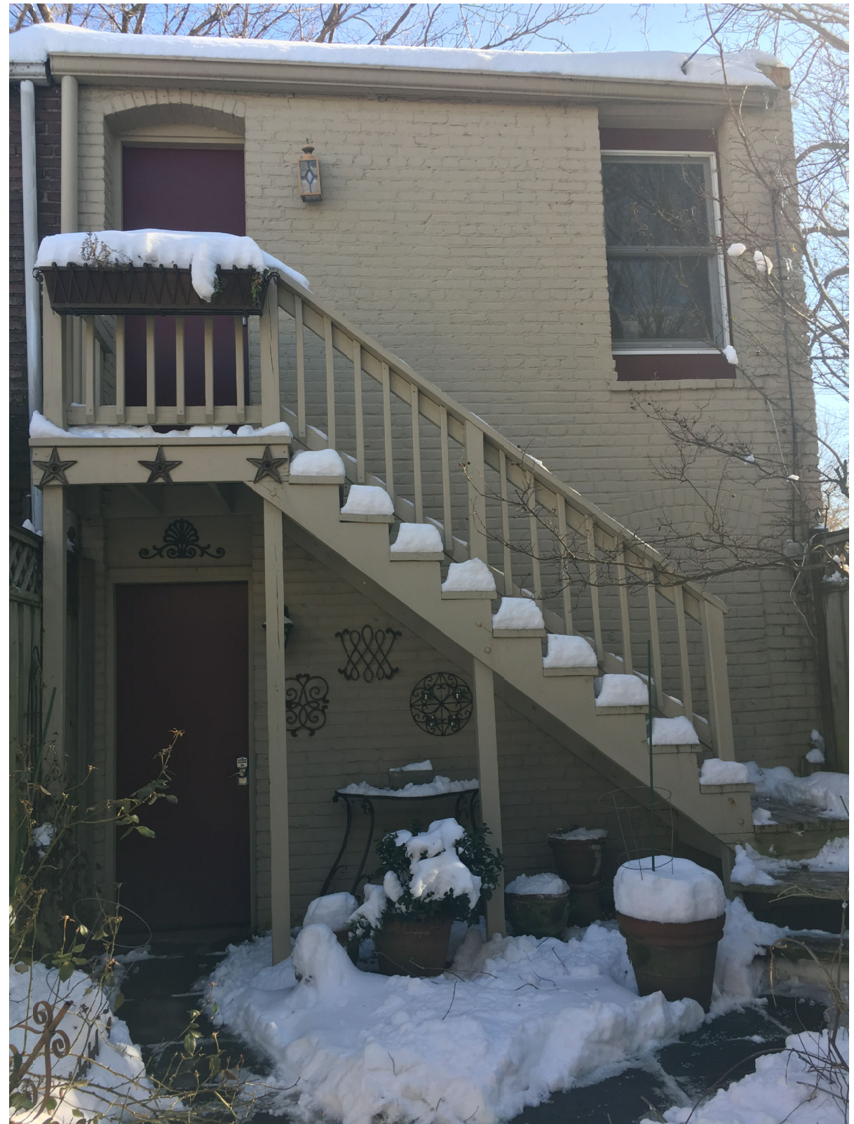
CARRIAGE HOUSE VIEW FROM REAR YARD
