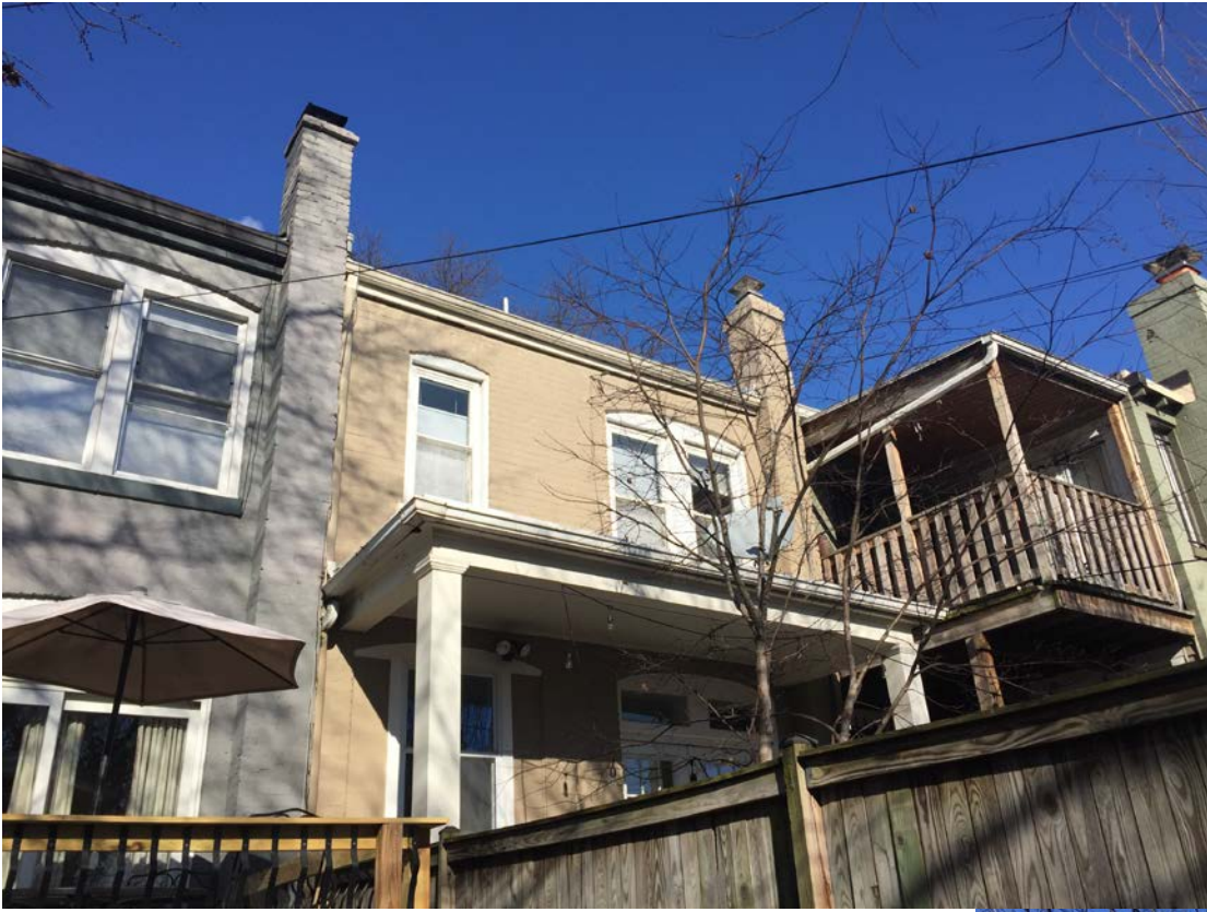
REAR FAÇADE, LOOKING EAST
