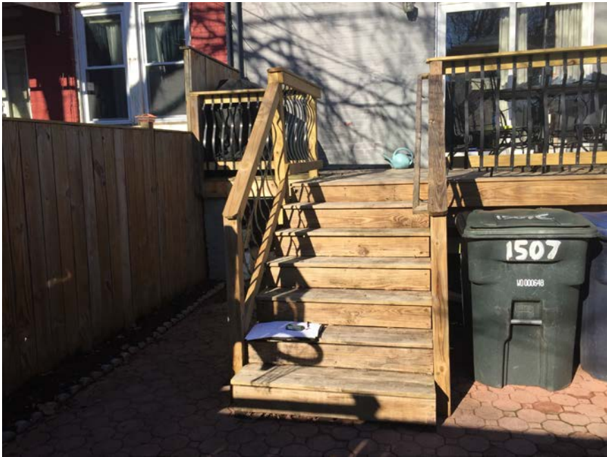
EXISTING DECK & STEPS TO GRADE
