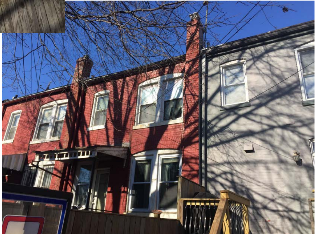
REAR FAÇADE, LOOKING WEST
