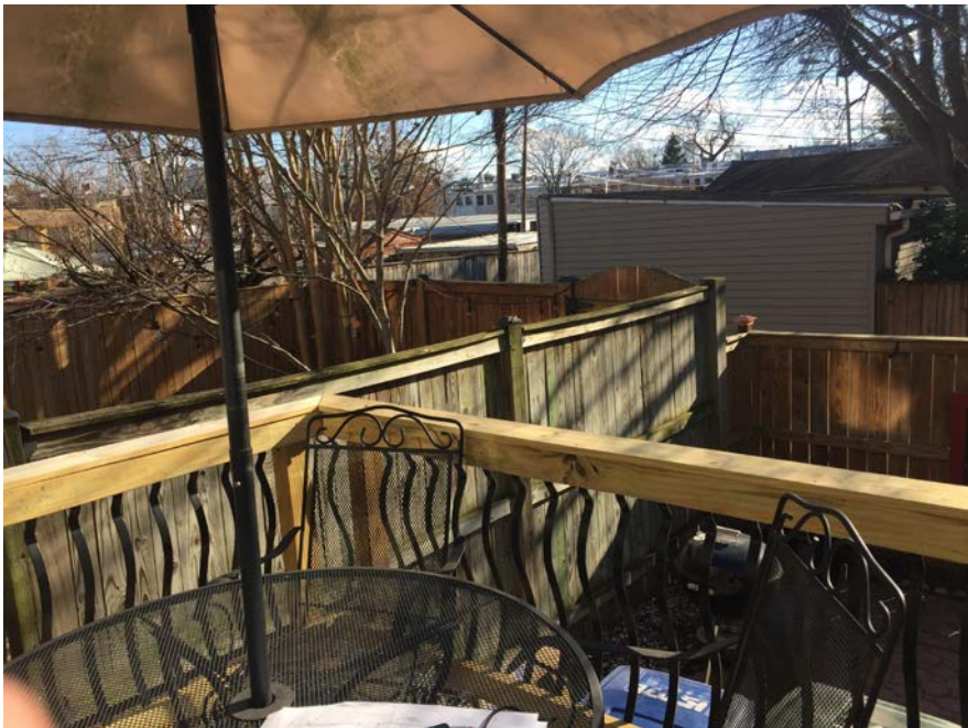
VIEW FROM EXISTING DECK, LOOKING EAST
