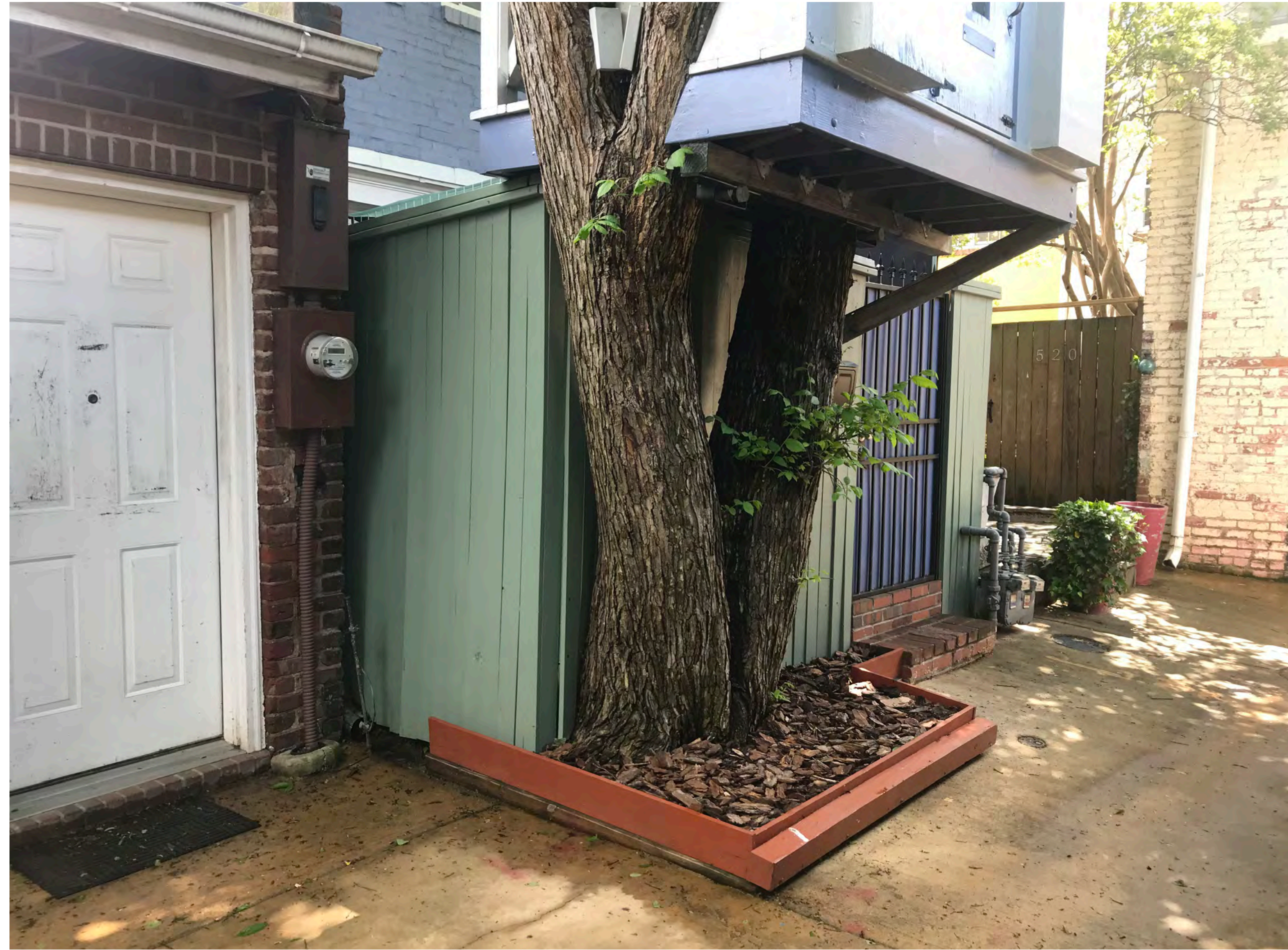
View of the Archibald Walk Entrance
