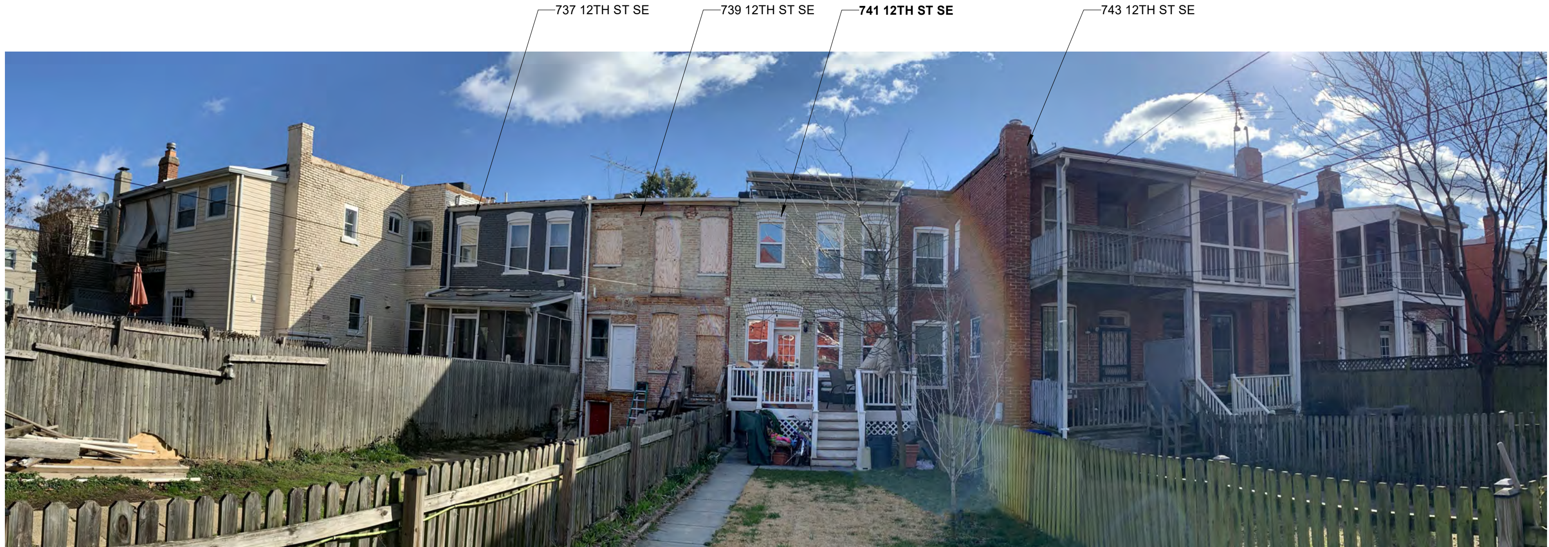
REAR FACADE PANORAMA FROM BACKYARD
