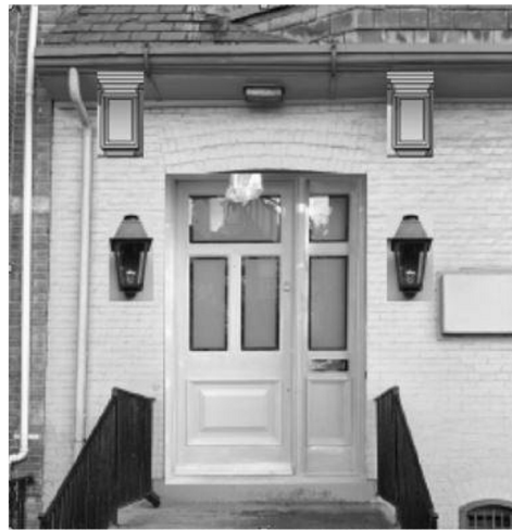
3. FRONT ENTRY AND LIGHTING
