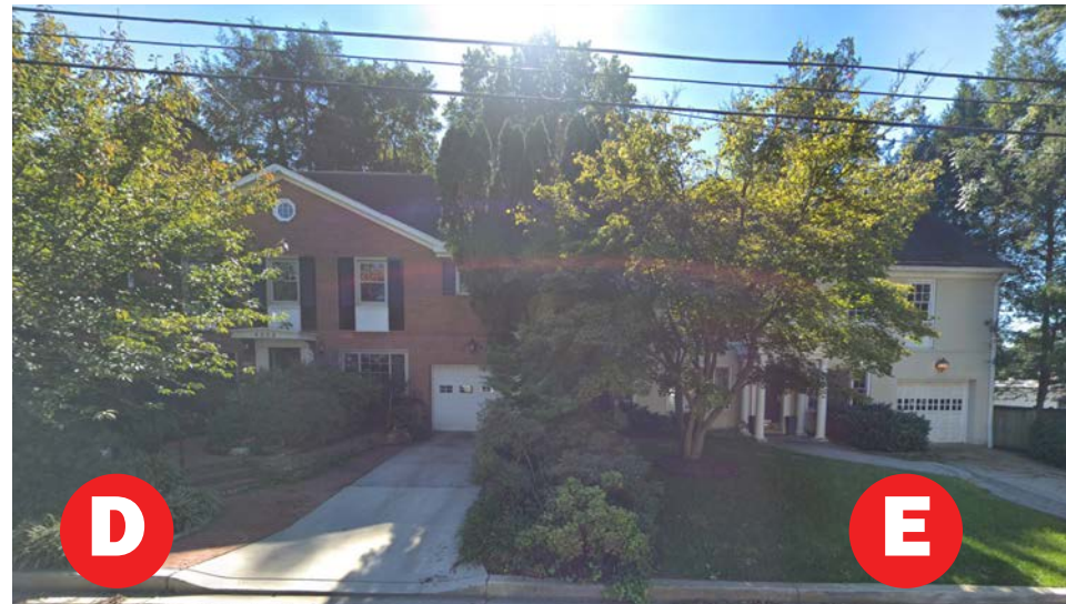
4808 V STREET NW (D-LEFT) & 4812 V STREET NW (E-RIGHT)
