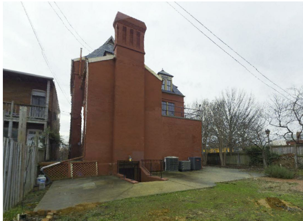
REAR YARD LOOKING SOUTHWEST
