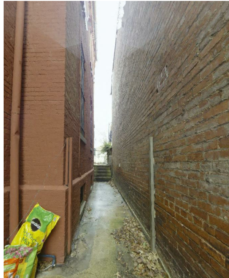
EAST SIDE YARD
