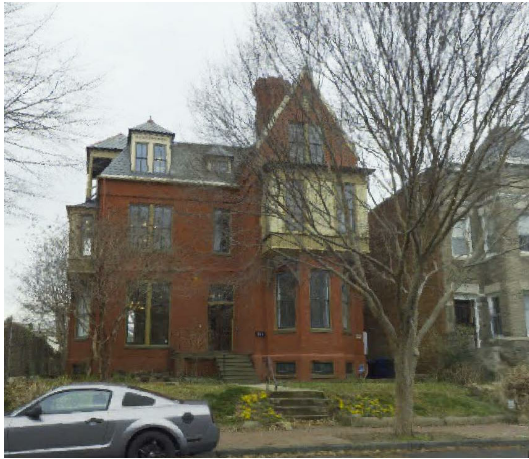
T STREET LOOKING NORTHEAST
