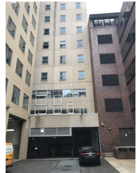
ALLEY LOOKING SOUTH
