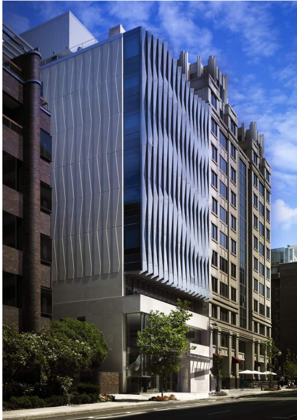
AT RISK WINDOWS ON NYU DC BUILDING
