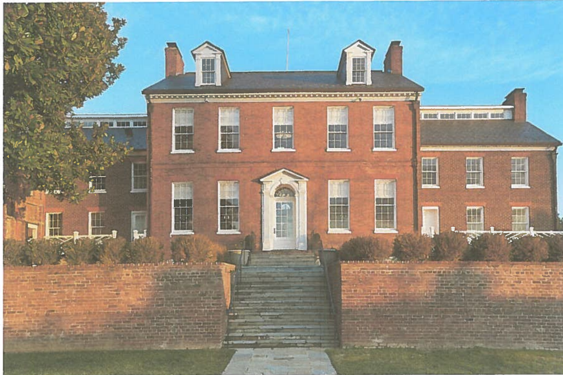
Rear Facade facing south to Arlington, VA
