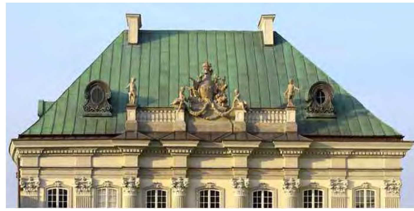
COPPER ROOF REFERENCE
