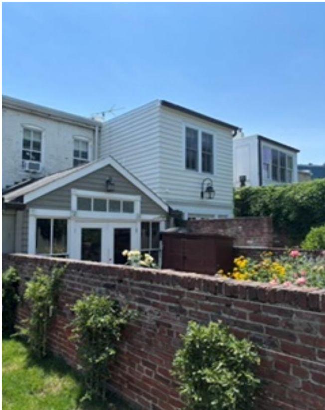
Rear view of 3313, 3315, 3317 P Street NW.
