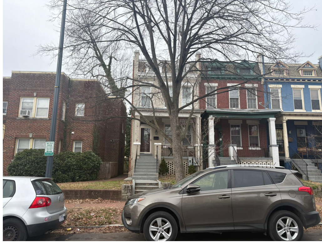
VIEW ACROSS 5 TH STREET NE
