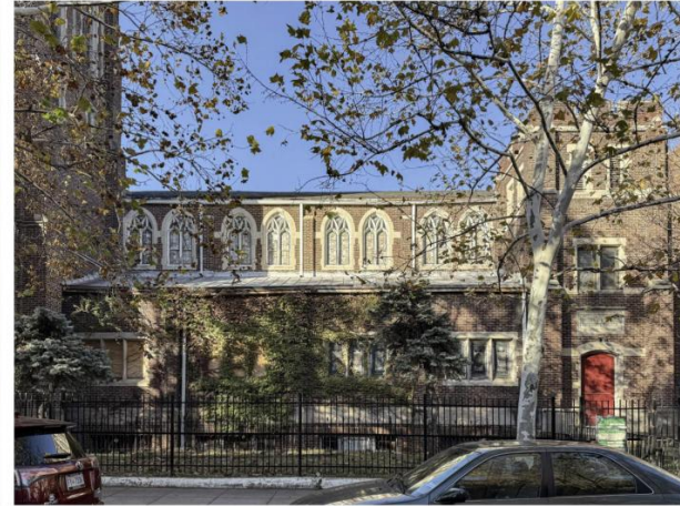
3. COLUMBIA RD NW - VIEW OF 1914 ADDITION
