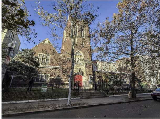
1. COLUMBIA RD NW - VIEW OF BELL TOWER
