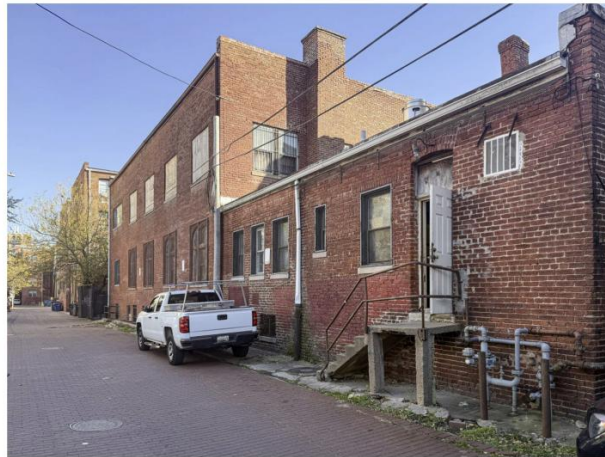
5. PUBLIC ALLEY - NW CORNER
