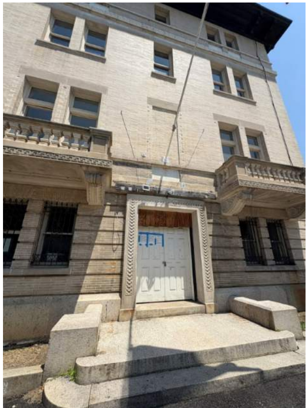
EXISTING ENTRY CONDITION
