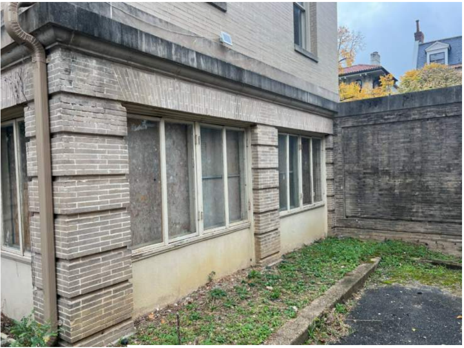
AREA OF PROPOSED GARAGE DOORS
