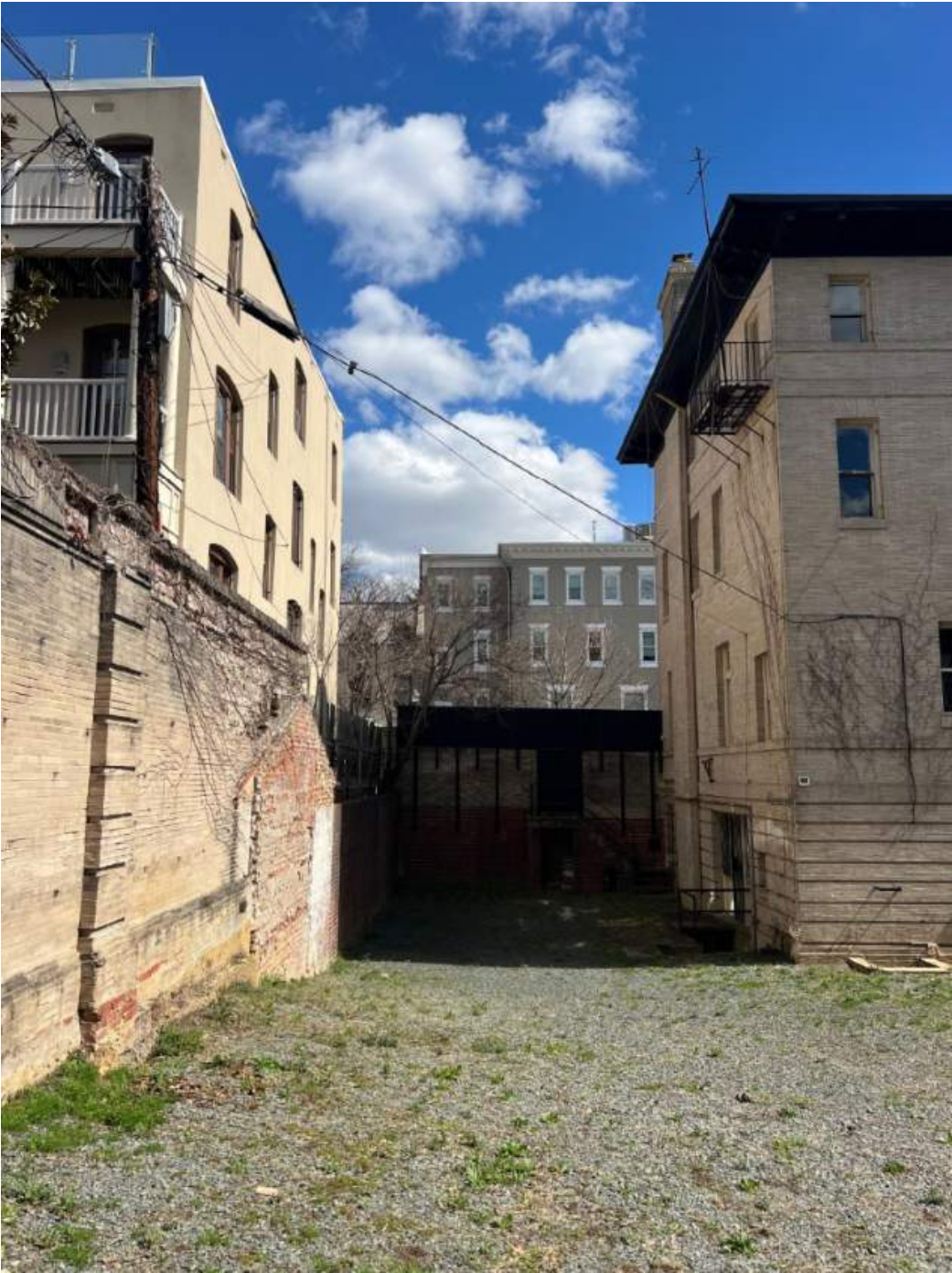
NEIGHBORING BUILDING RELATIONSHIP ON 22ND ST., NW
