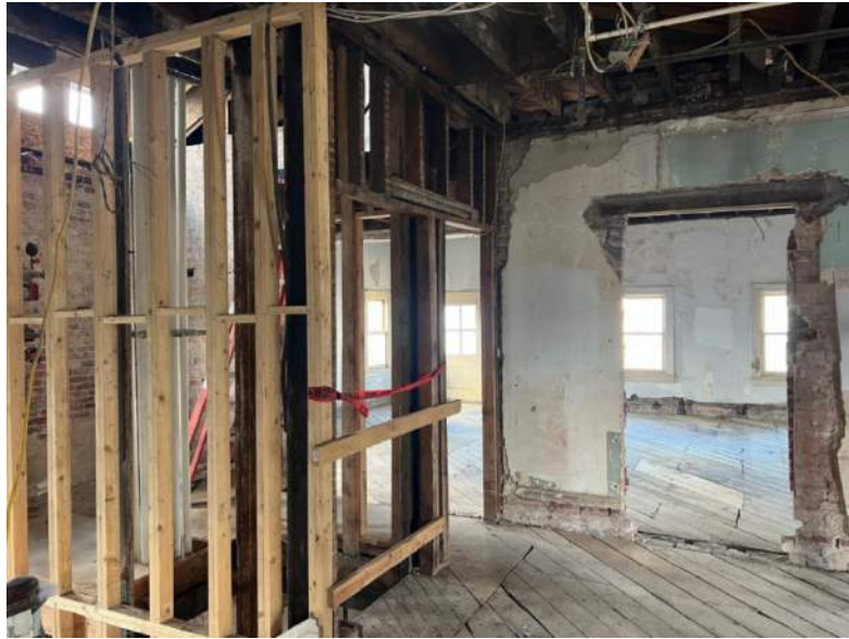
3RD FLOOR STAIR HALL FACING NORTH
