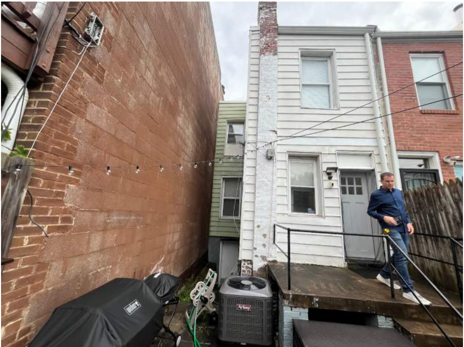
4. VIEW LOOKING E FROM REAR YARD OF 443 17TH ST SE
