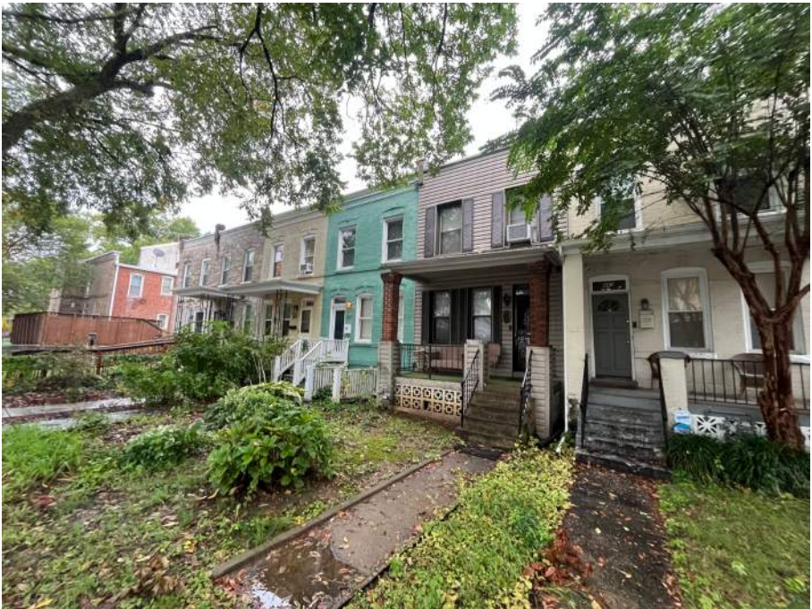
2. VIEW LOOKING S FROM FRONT YARD OF 443 17TH ST SE
