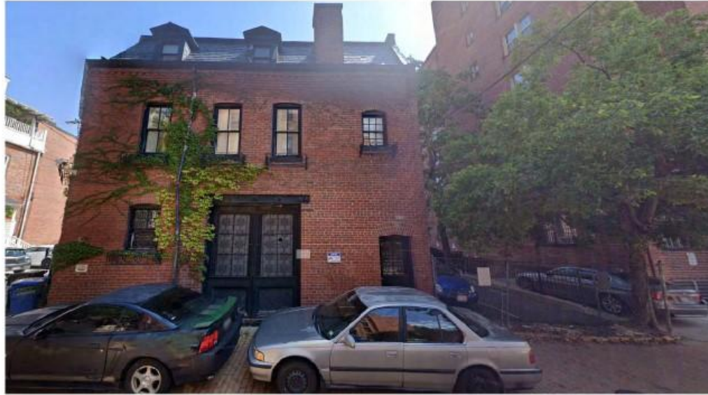
2 EXISTING VIEW TO THE WEST SCALE: NONE
