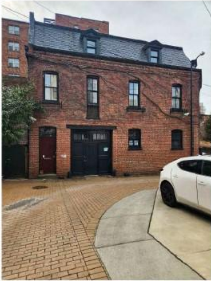
1 EXISTING VIEW TO THE NORTH SCALE: NONE
