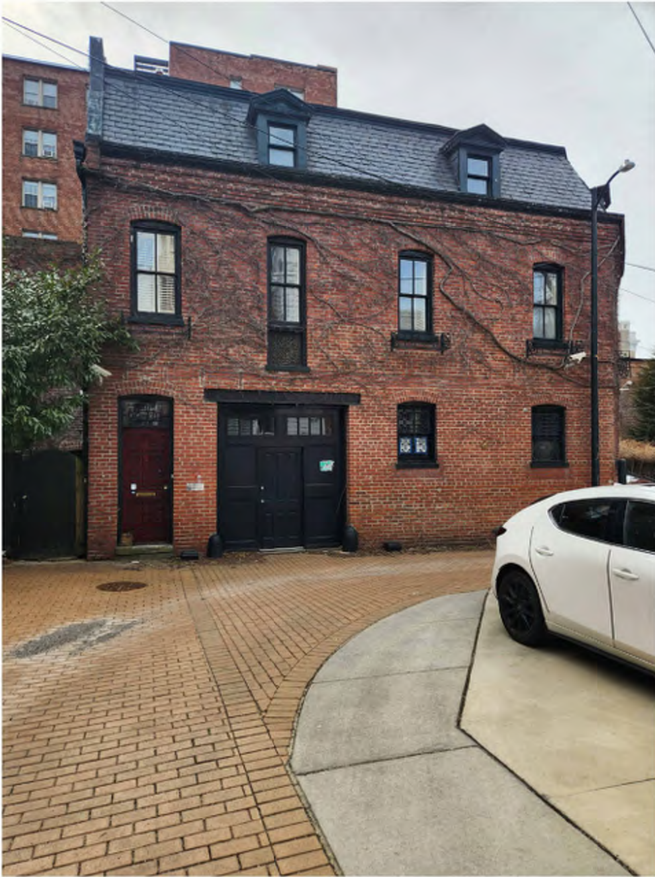
1 EXISTING VIEW TO THE NORTH SCALE: NONE
