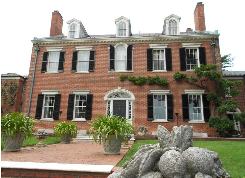
South Elevation Looking from Rear Door
