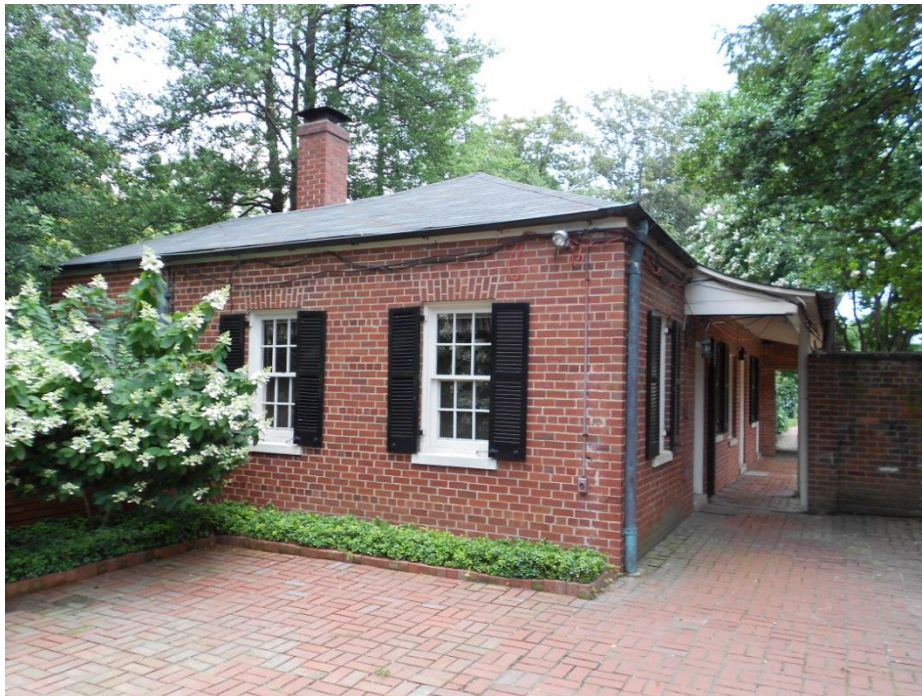
View Looking North at Staff Offices along West Property Line at 28th Street, N.W.
