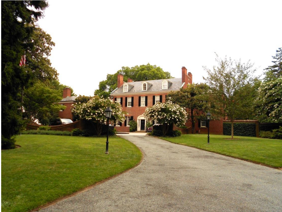
North Elevation Driveway to Courtyard
