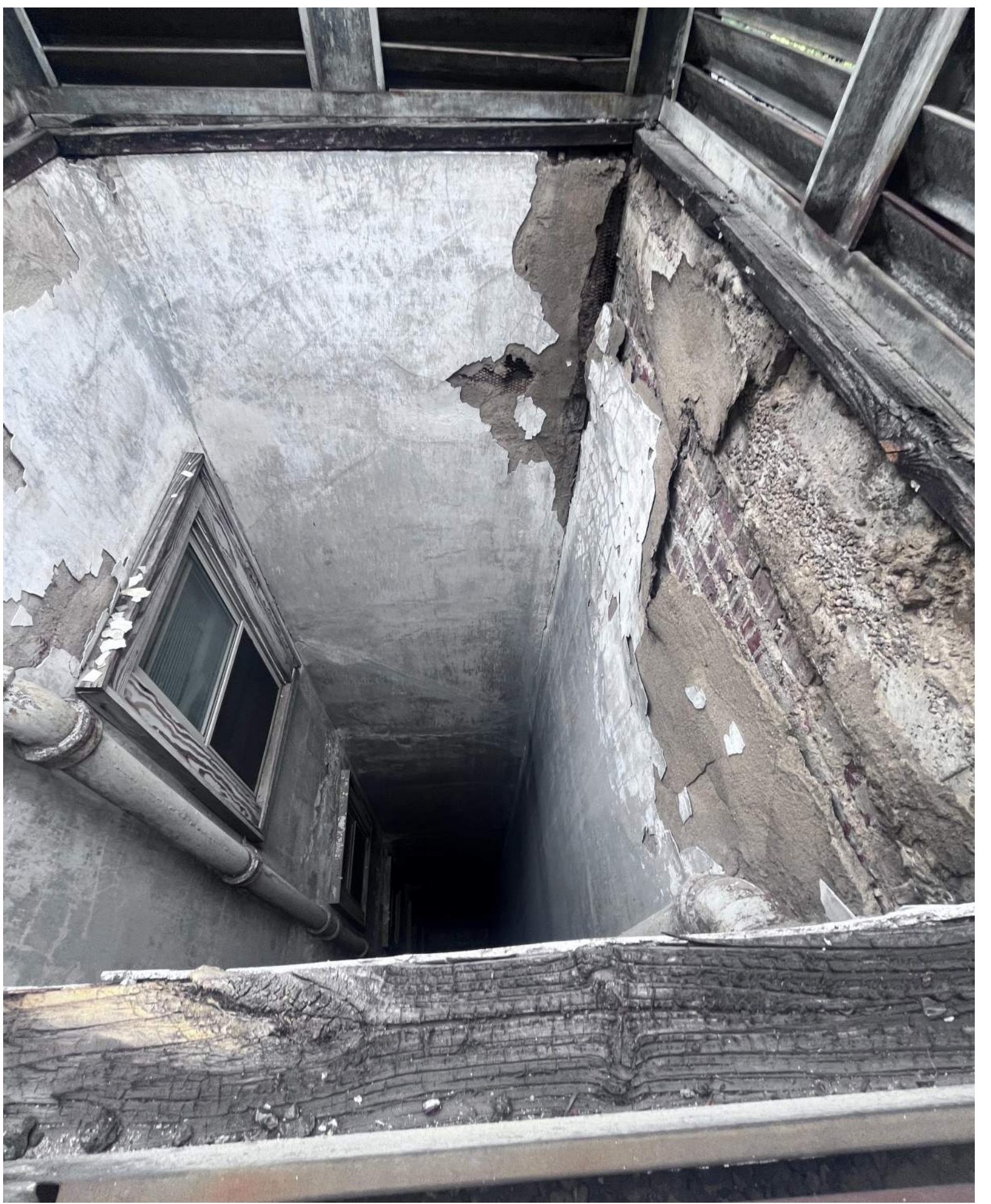
10. REPAIR VENTILATION SHAFT WALLS AND WATER INTRUSION ISSUE
