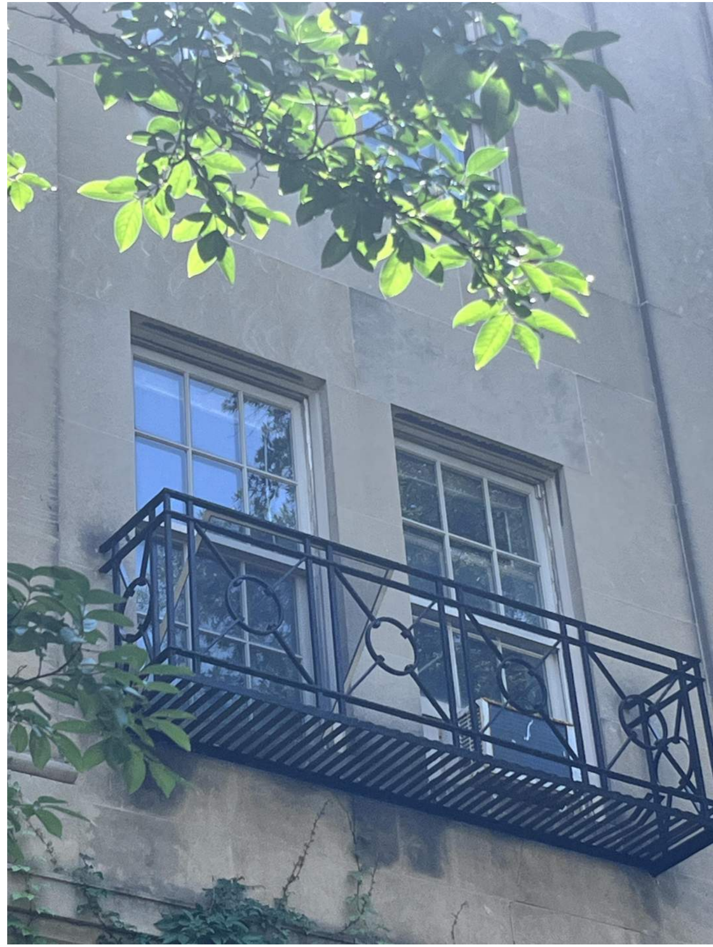
2. LIMESTONE CLEANING AND REPAIR HISTORIC FACADE
