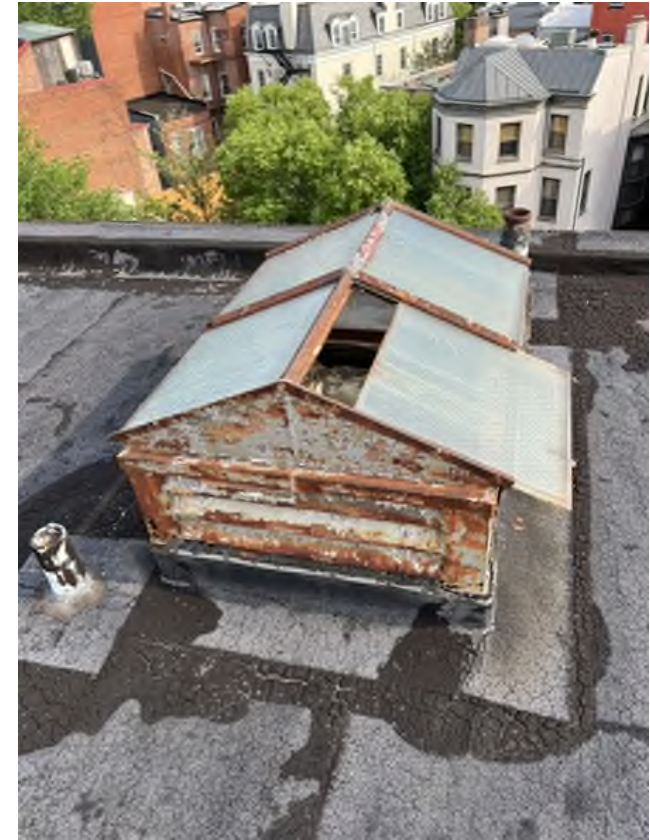
Deteriorated skylight
