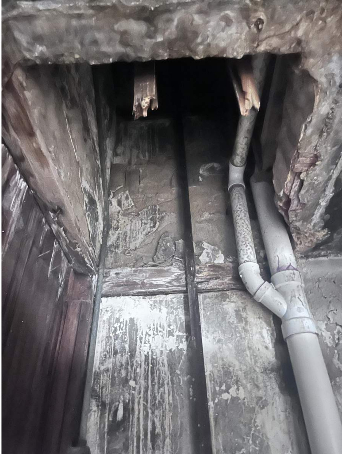
5. ABANDONED DUMBWAITER SHAFT
