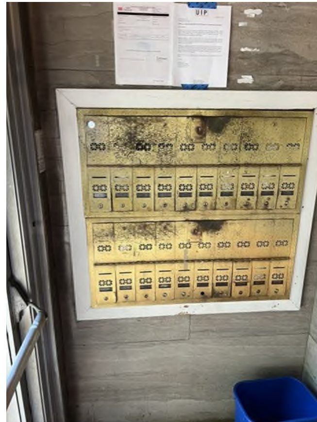
Rusting resident mailbox
