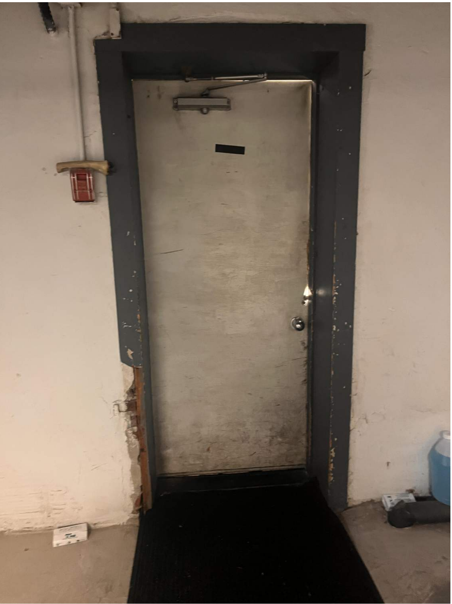
9. REPLACE DAMAGED AND FRAMES THROUGHOUT, NON-RATED DOORS & FRAMES AT RATED WALLS WITH NEW CODE-COMPLIANT FIRE-RATED DOORS, FRAMES & CLOSERS, ALL LEVELS.
