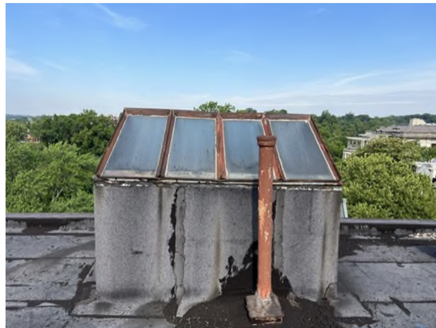
Deteriorated skylight
