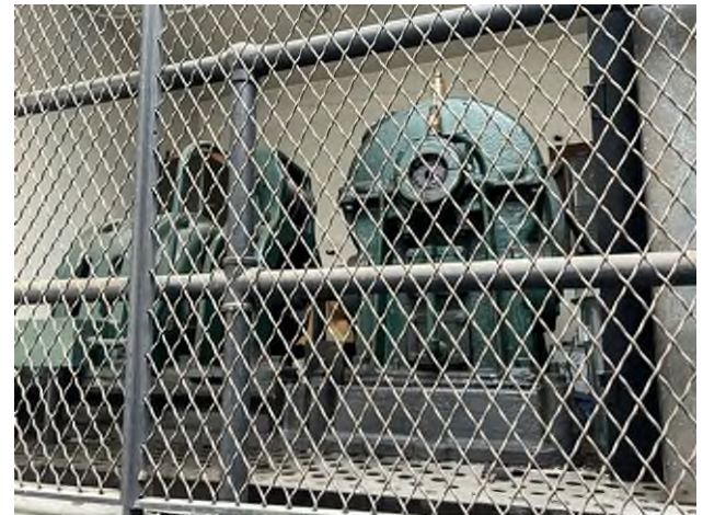
Extremely dated elevator system – proposed full system update
