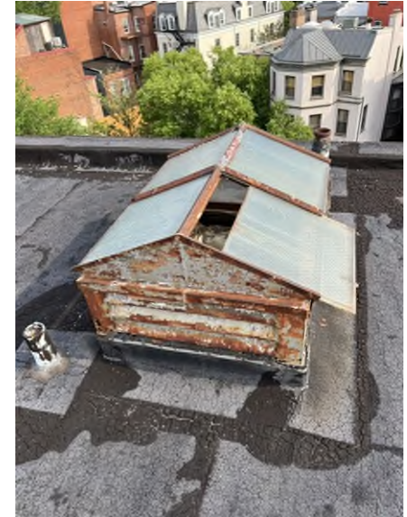
Deteriorated skylight
