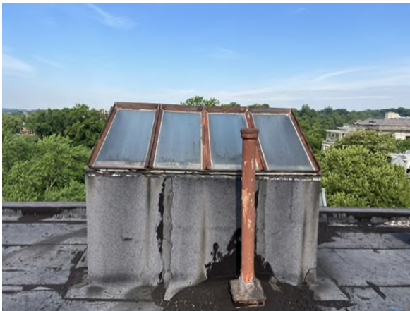
Deteriorated skylight
