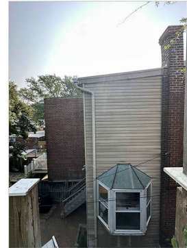
VIEW FROM 2ND LEVEL PORCH LOOKING EAST
