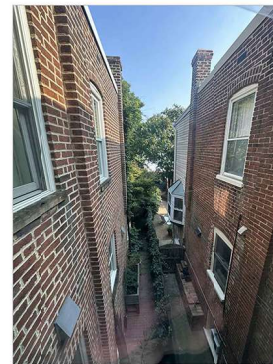
VIEW OF DOGLEG CONDITION FROM SECOND LEVEL
