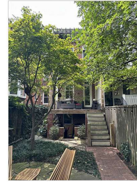
REAR FACADE: VIEW FROM YARD
