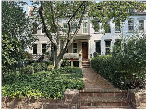
FRONT FACADE: VIEW FROM SIDEWALK
