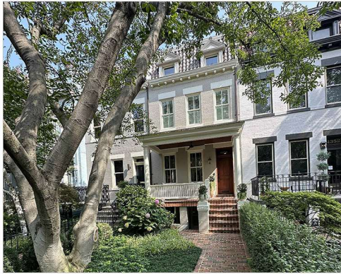
FRONT FACADE: VIEW FROM YARD
