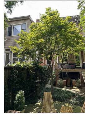
REAR FACADE: LOOKING EASTWARD
