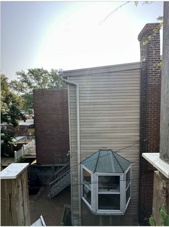
VIEW FROM 2ND LEVEL PORCH LOOKING EAST
