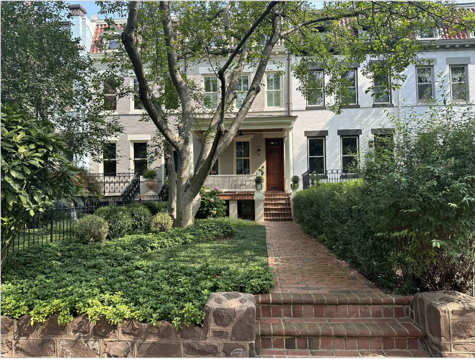
FRONT FACADE: VIEW FROM SIDEWALK
