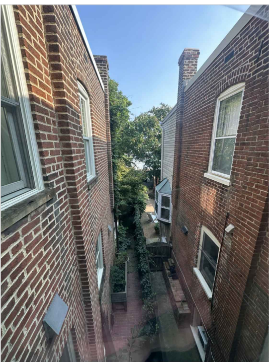
VIEW OF DOGLEG CONDITION FROM SECOND LEVEL
