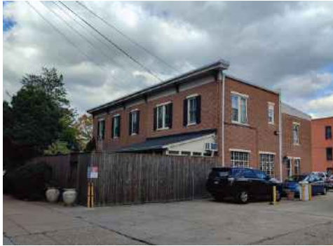
3 | St Joseph's Rectory Addition
