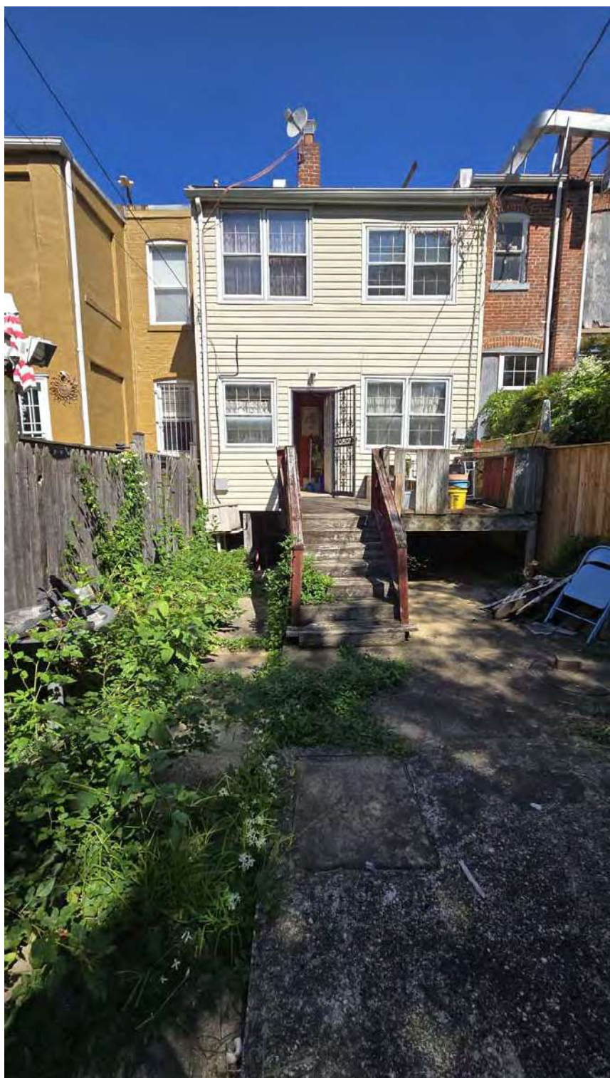
EXISTING REAR WALL
