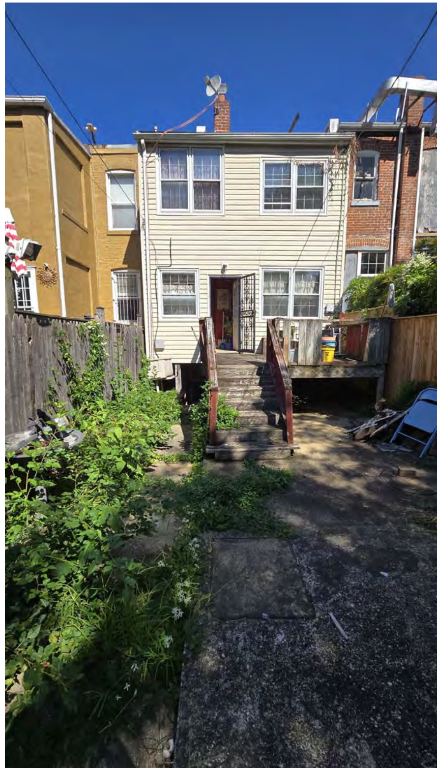
EXISTING REAR WALL
