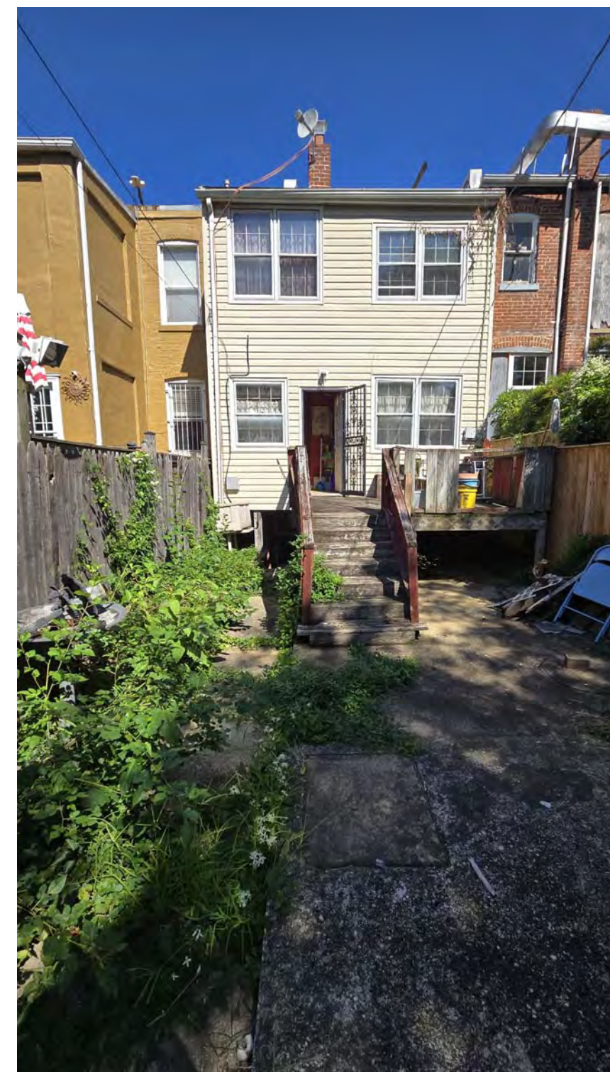
EXISTING REAR WALL
