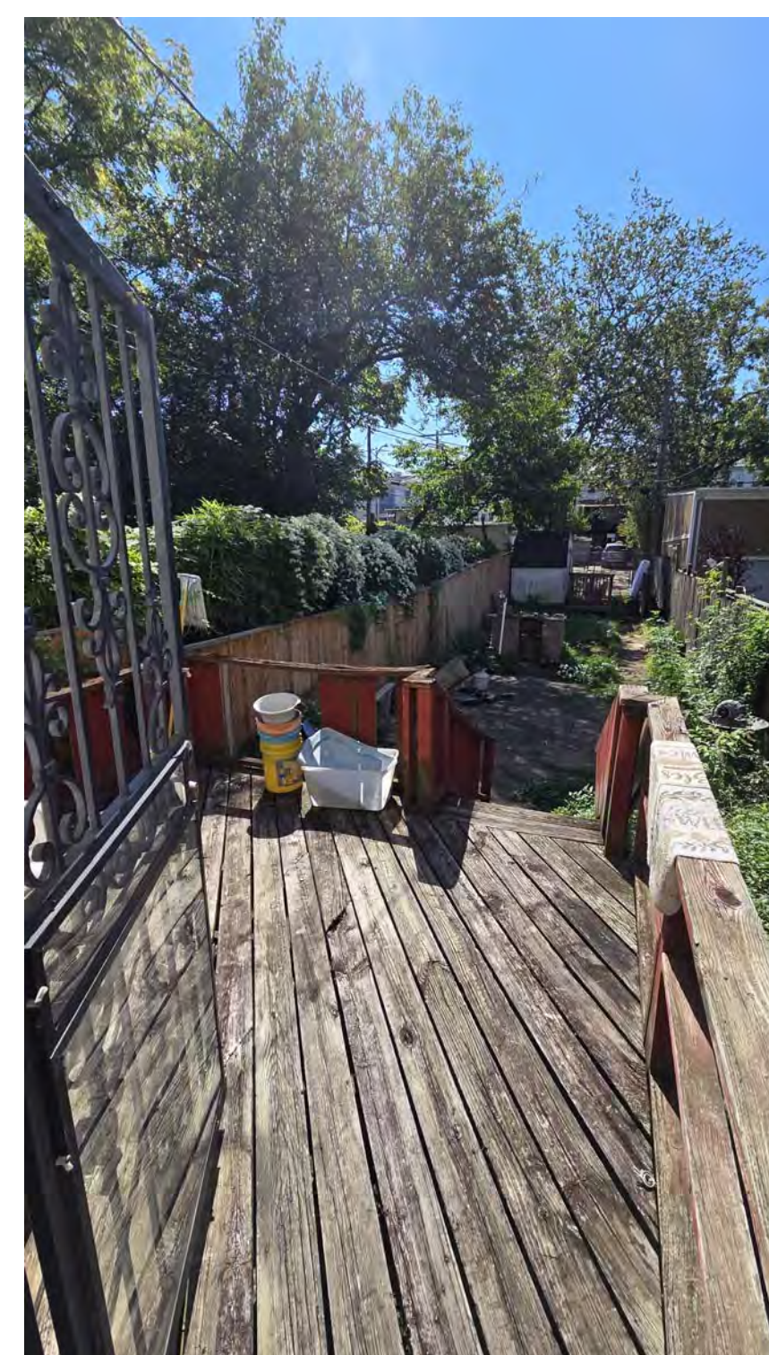
VIEW TOWARDS REAR ALLEY
