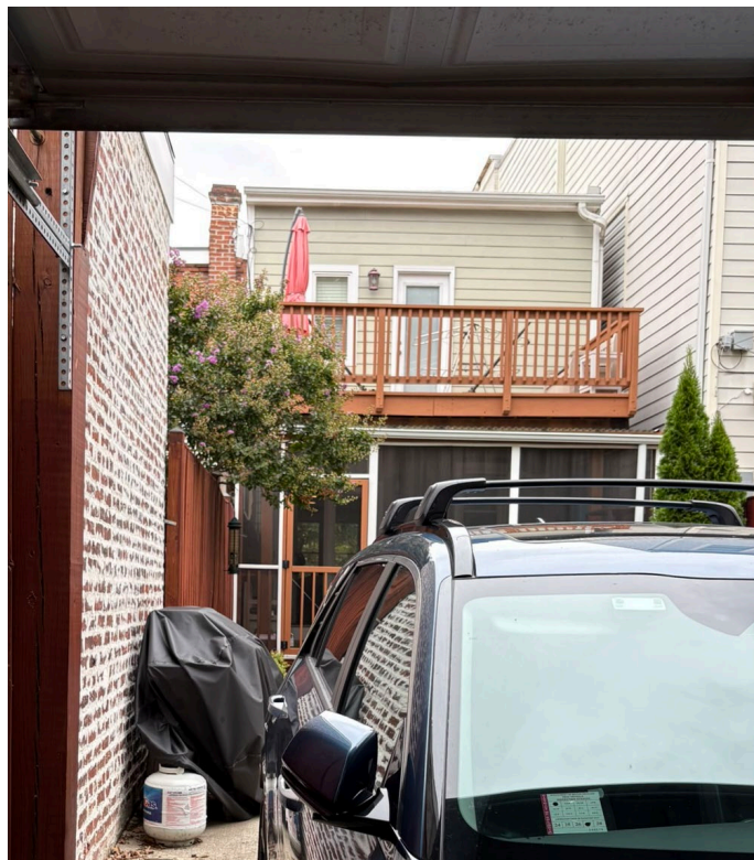
EXISTING REAR FAÇADE, FROM ALLEY
