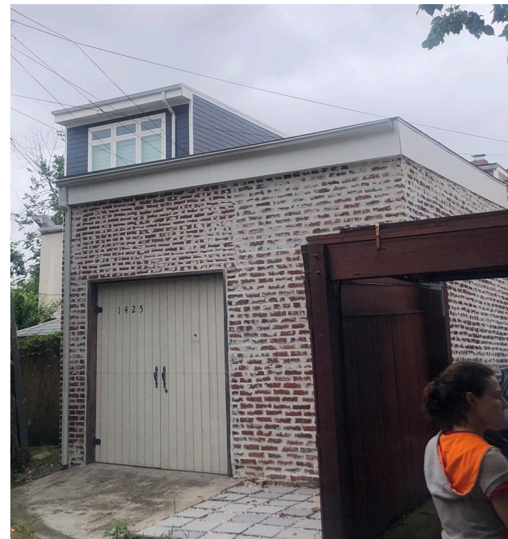
EXISTING GARAGE @ 1425 D STREET SE
