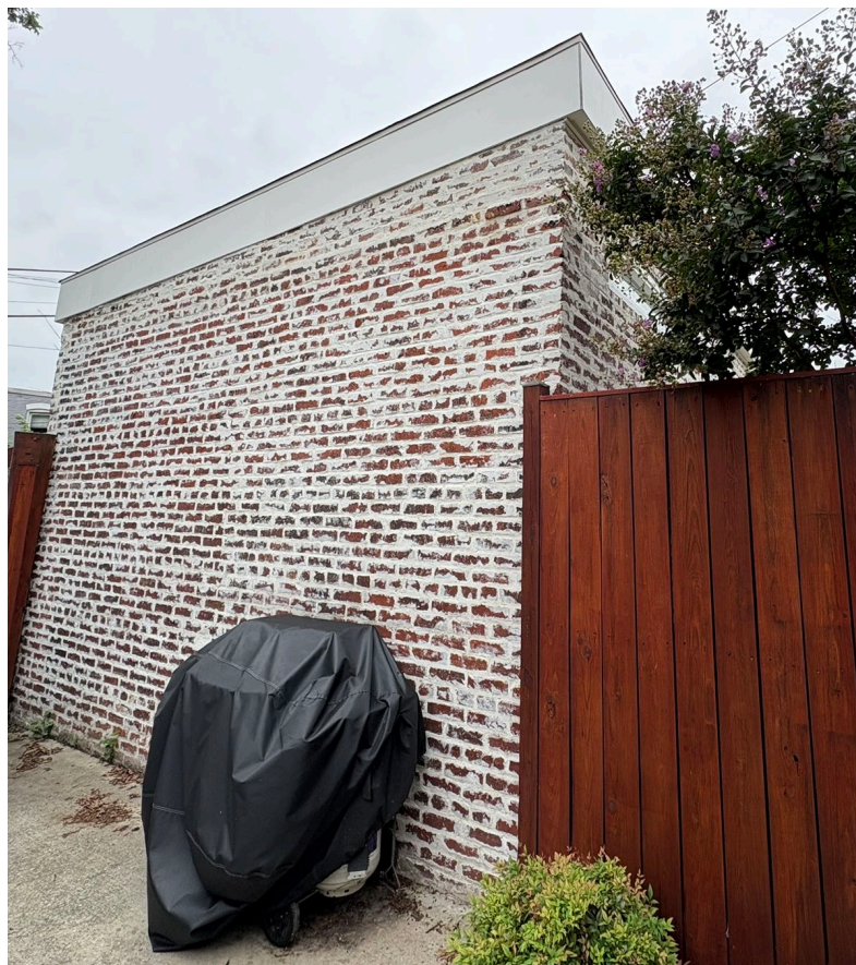
EXISTING GARAGE @ 1425 D STREET SE
