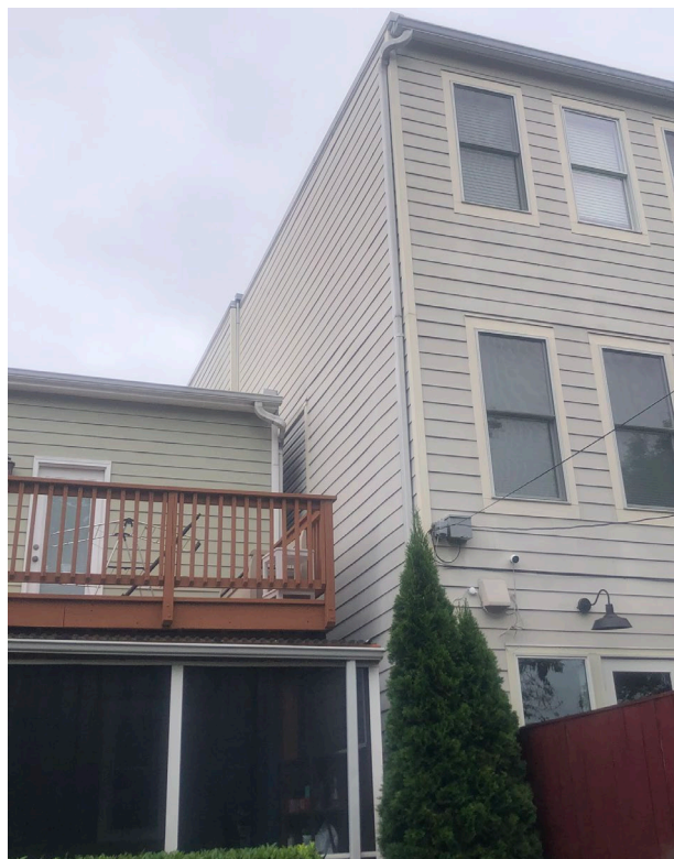
EXISTING REAR FAÇADE, LOOKING EAST
