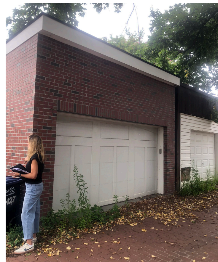
EXISTING GARAGE @ 1429 D STREET SE (VIEW FROM ALLEY)
